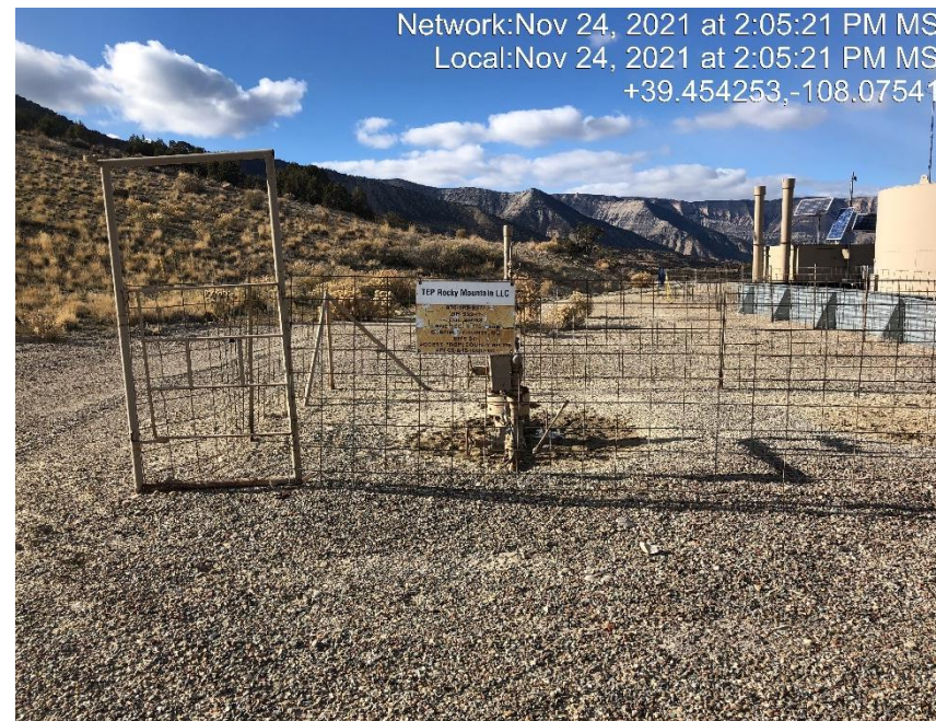
Photo #5260 Wellhead sign weathered and not legible.
