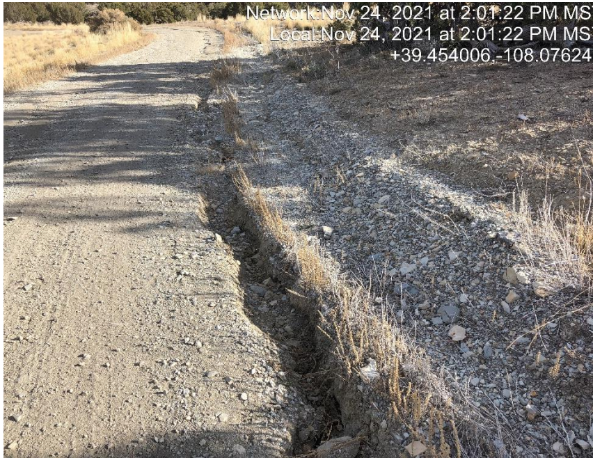
Photo #5256 Insufficient velocity checks in ditches.
