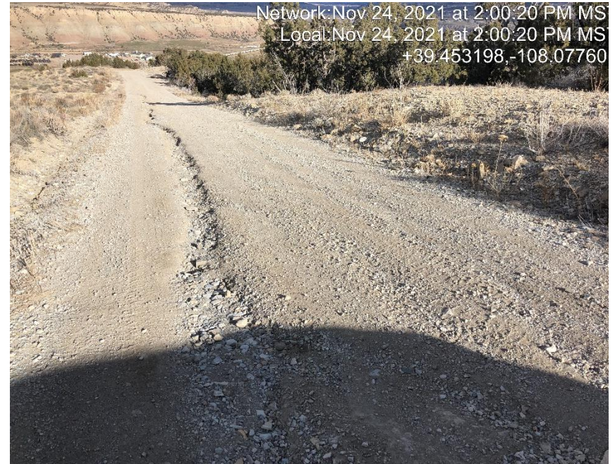
Photo #5255 Rill erosion occurring in access road.
