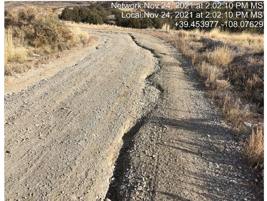
Photo #5257 Rill erosion occurring in access road.
