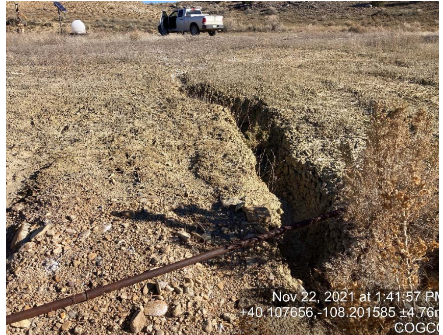
Erosion on fill slope /sediment migration from pad
