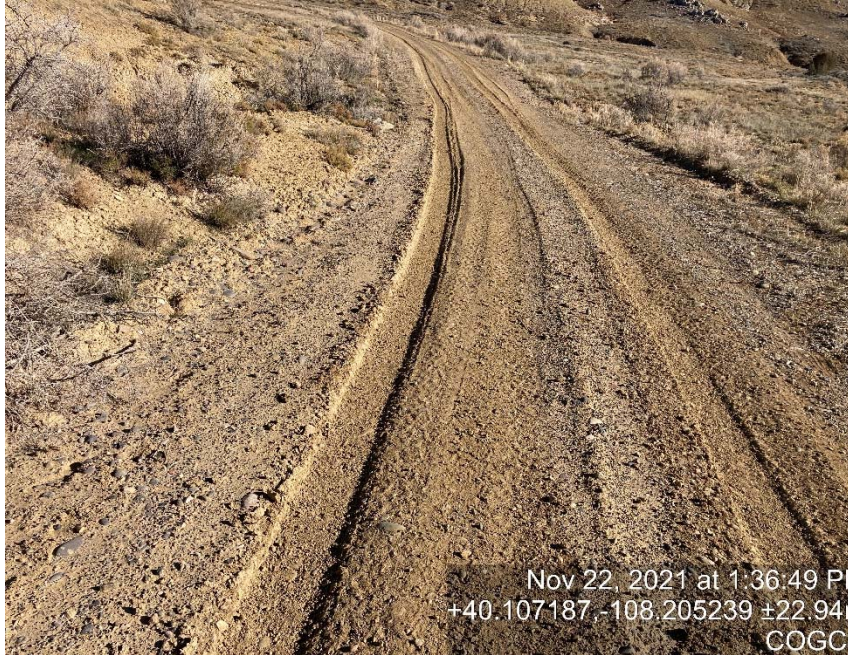
Lack of stabilization/compaction
