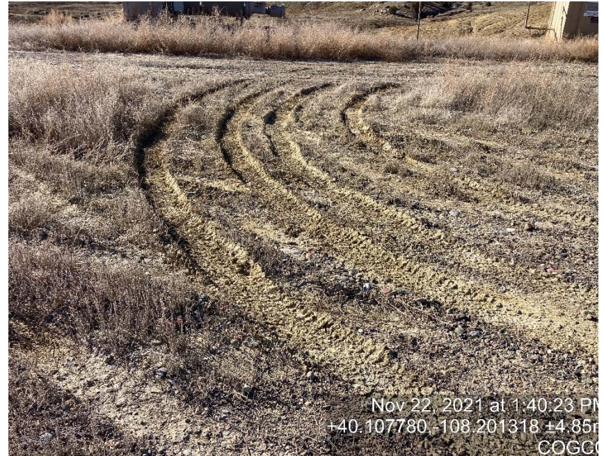
Lack of stabilization/compaction
