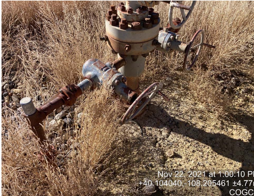
Lack of Braden head access
