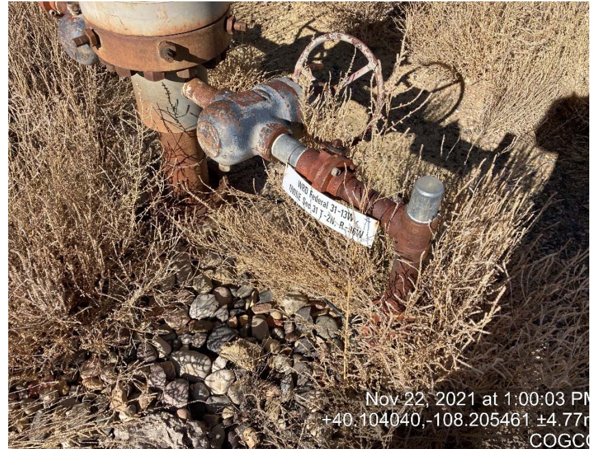
Lack of Braden head access
