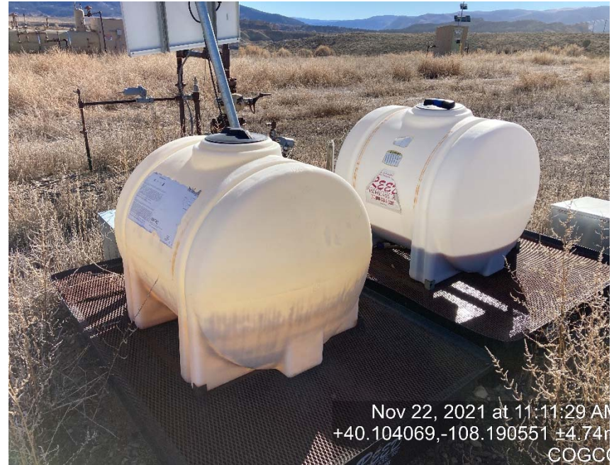
Chemical tanks lacking labeling
