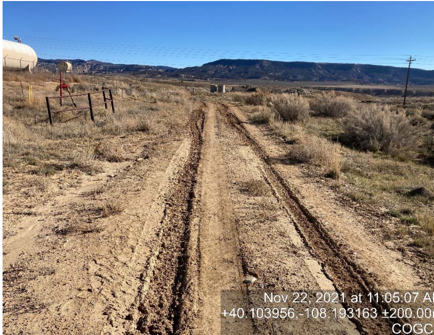
Lack of stabilization/compaction
