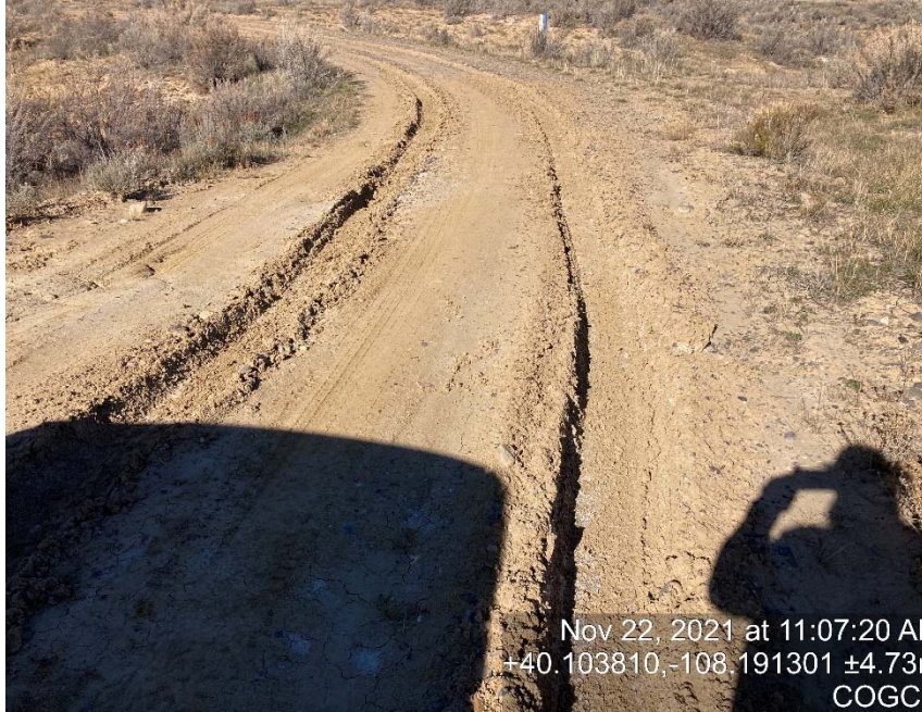
Lack of stabilization/compaction
