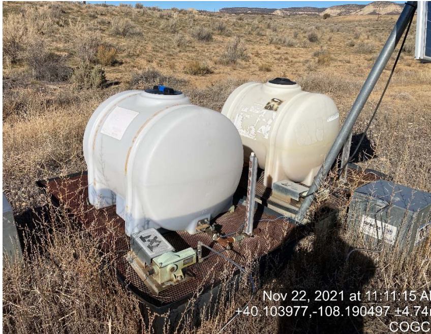
Chemical tanks lacking labeling
