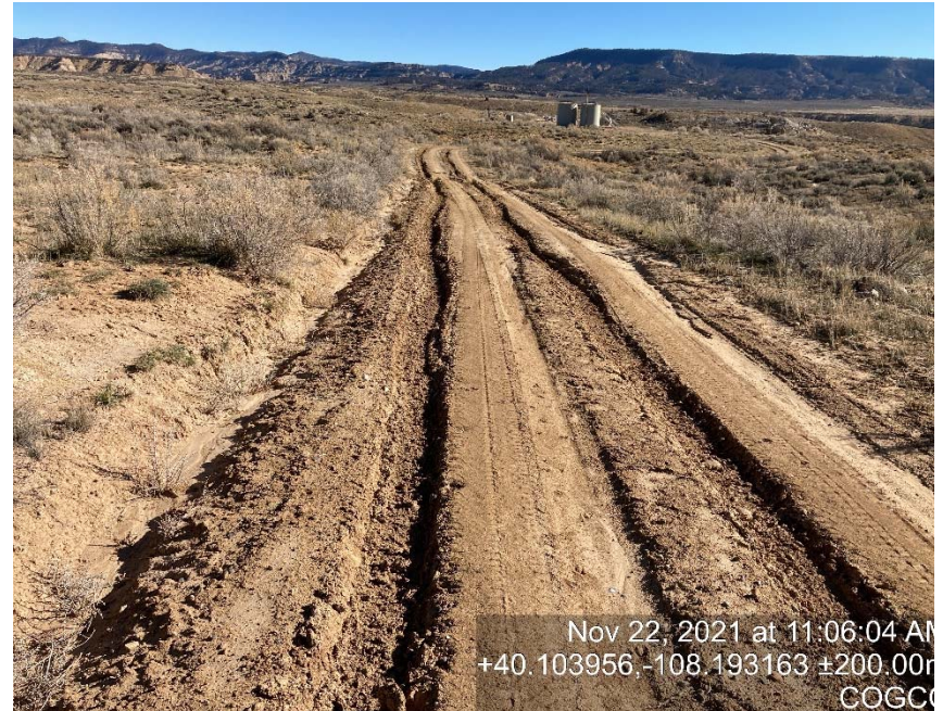
Lack of stabilization/compaction
