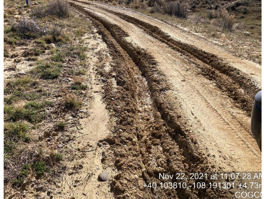
Lack of stabilization/compaction
