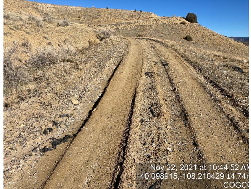
Lack of stabilization/compaction
