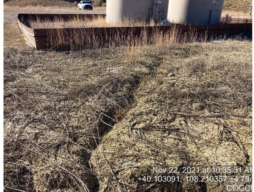
Erosion channels from location with sediment migration
