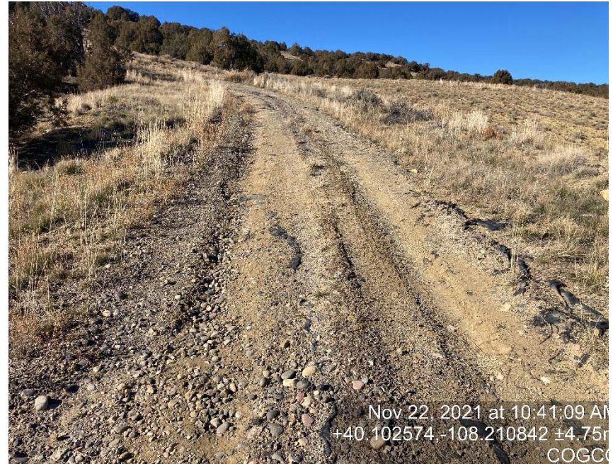
Lack of stabilization/compaction
