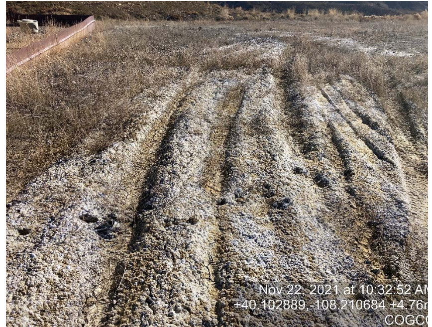
Lack of stabilization/compaction
