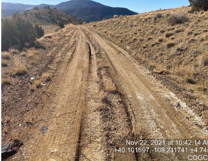
Lack of stabilization/compaction
