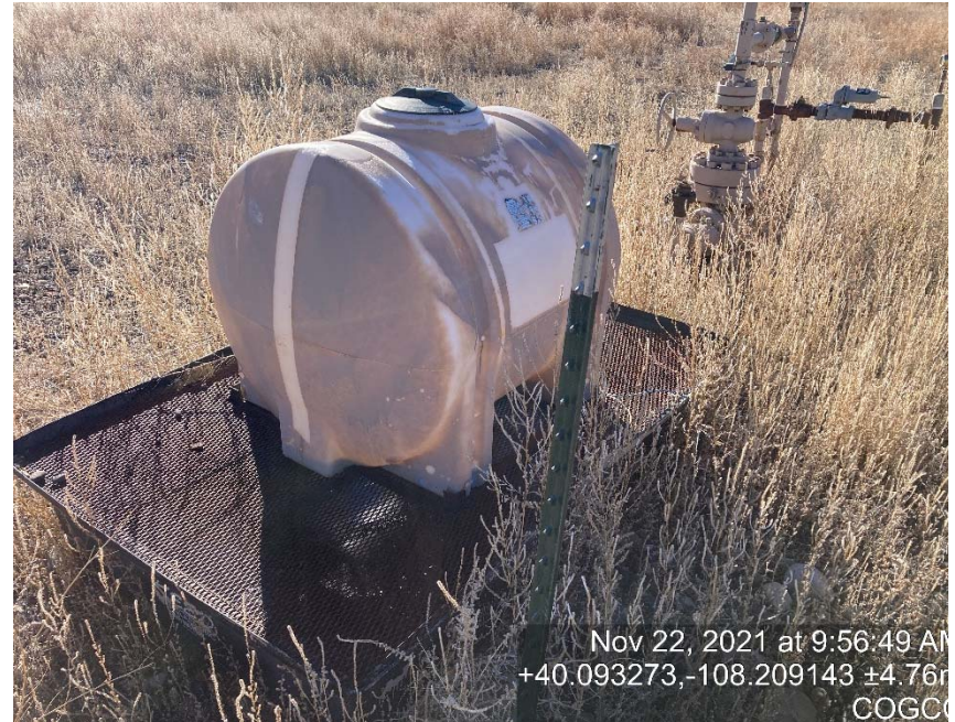
Unused chemical tank and containment
