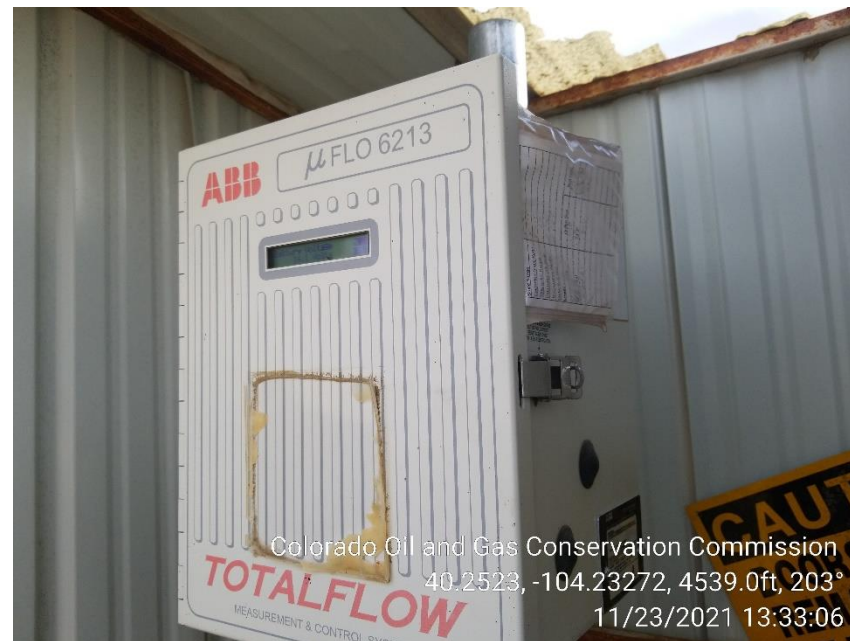
Photo 4 – Gas Meter – Calibration Card up to date
