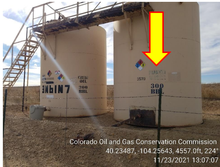
Photo 4 – Tank Battery – Produced Water Label is fading
