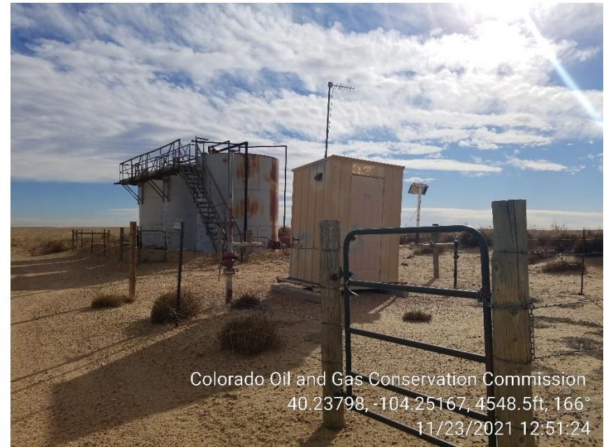
Photo 2 – Gas Engine House and Tank Battery
