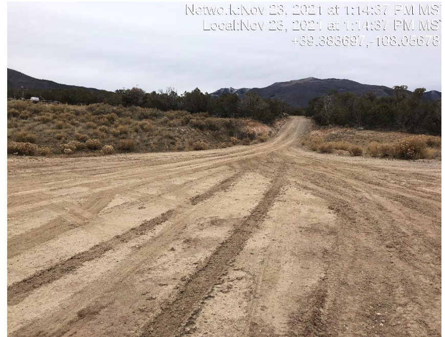
Photo #5240 No form of tracking BMP located at entrance to location.
