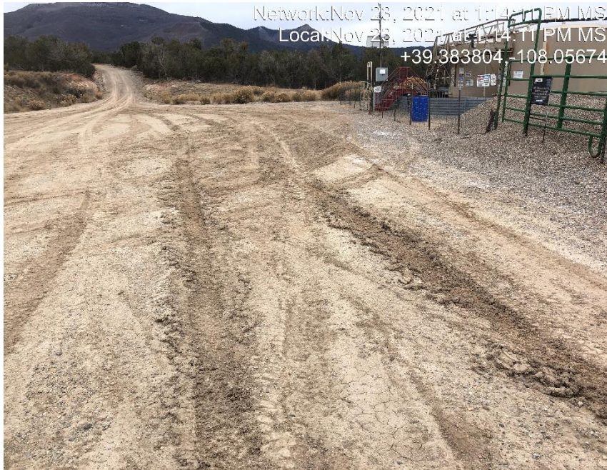
Photo #5239 location lacks stabilization.
