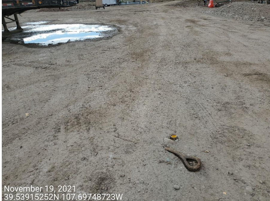
Photo 1: Anchors missing required markers.
