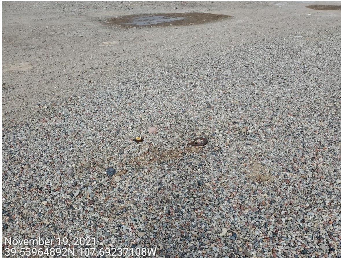
Photo 2: Anchor without required marker.
