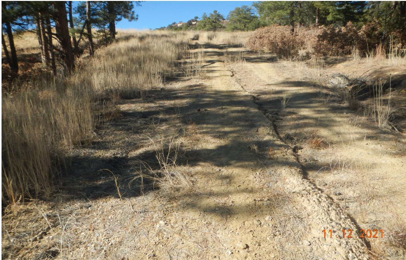
Photo 2. Facing northwest along the access road which has not been reclaimed. There are signs of erosion as the road ascends to the location.
