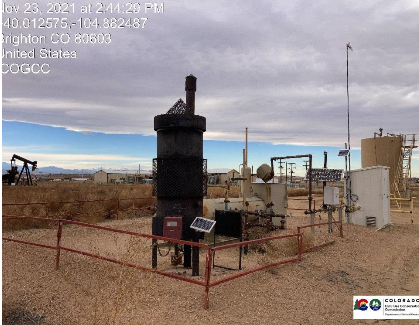
Pic 3 ECD, Separator, gas meter run
