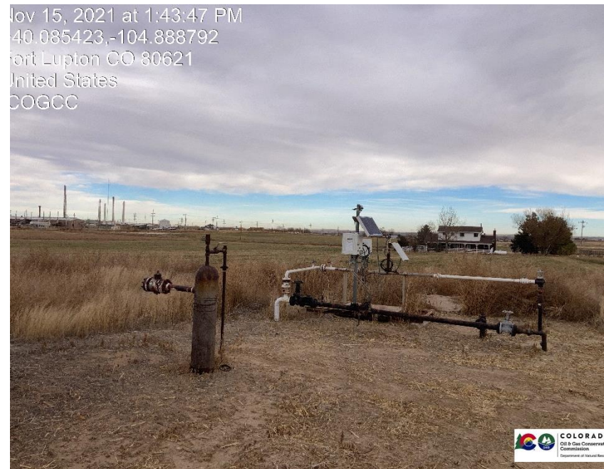
Pic 6 gas meter run / verticle vessel.
