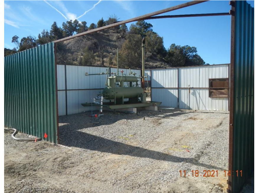
La Posta Canyon CDP separator within enclosure.
