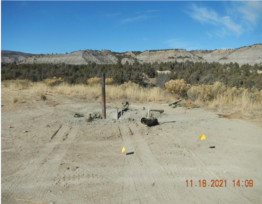
Jacques #2 well head has been cut off and PA marker welded onto casing.
