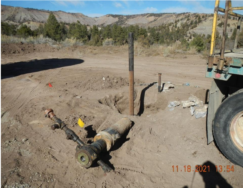
La Posta Canyon #2 cut off well head and PA marker.
