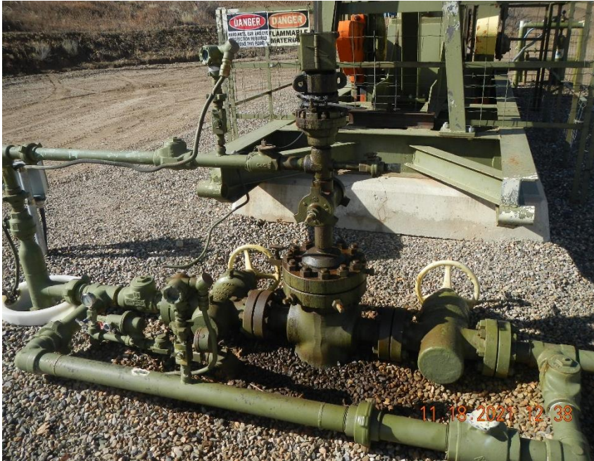
Southern Ute #5-7 well head. Well head and surrounding area are stained and wet.
