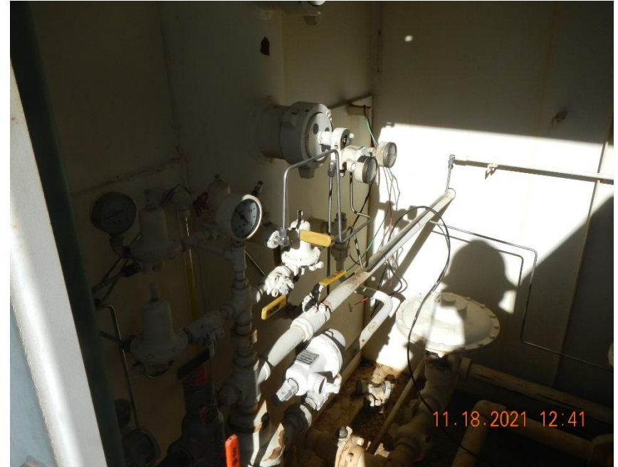
Audible leak from valve in separator shack during this inspection.
