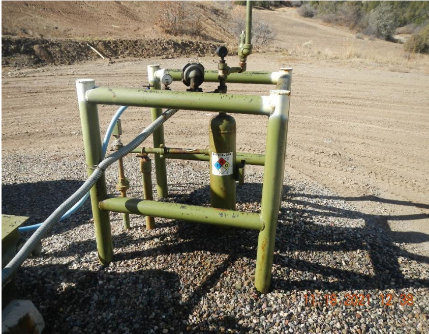
Wet and stained area near drop out tank.
