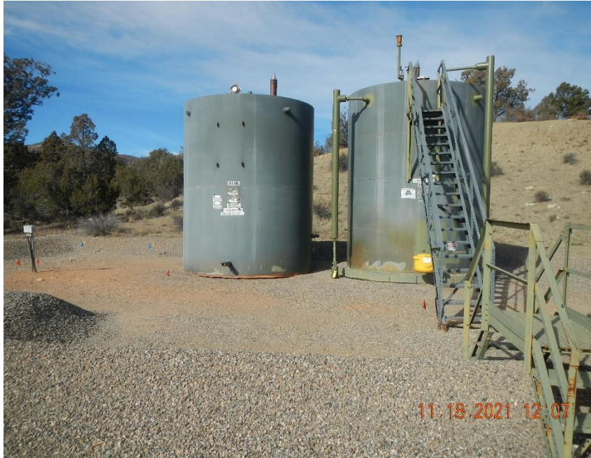
Thief hatch is open on left AST. Signs and placards are not compliant with Rule 605.h.
