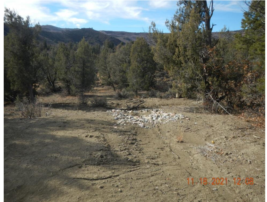
Rip rap BMP has filled in with sediment.
