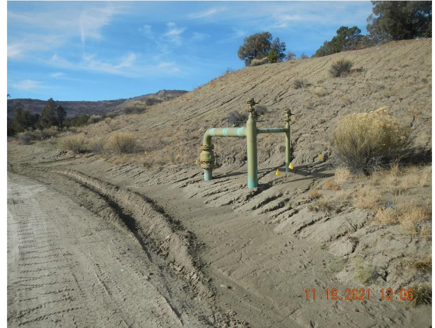
Sediment is being transported onto location from the cut slope.
