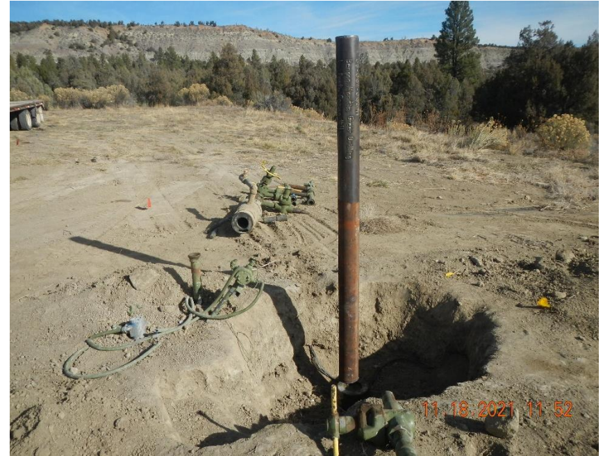
Close up of cut off well head and PA marker.
