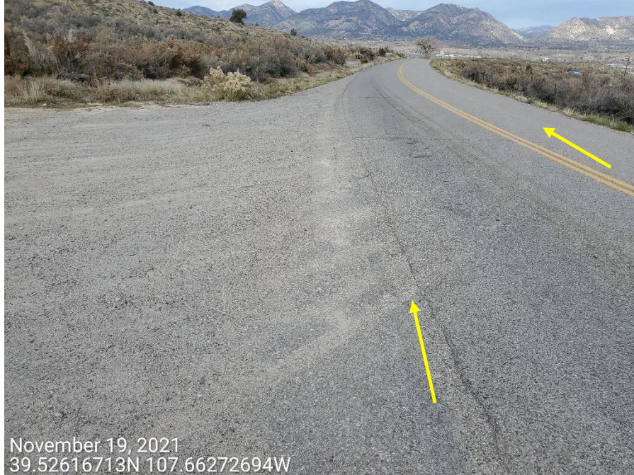
Photo 9: Continued from photo 8. Photo shows sediment transport onto the county road.
