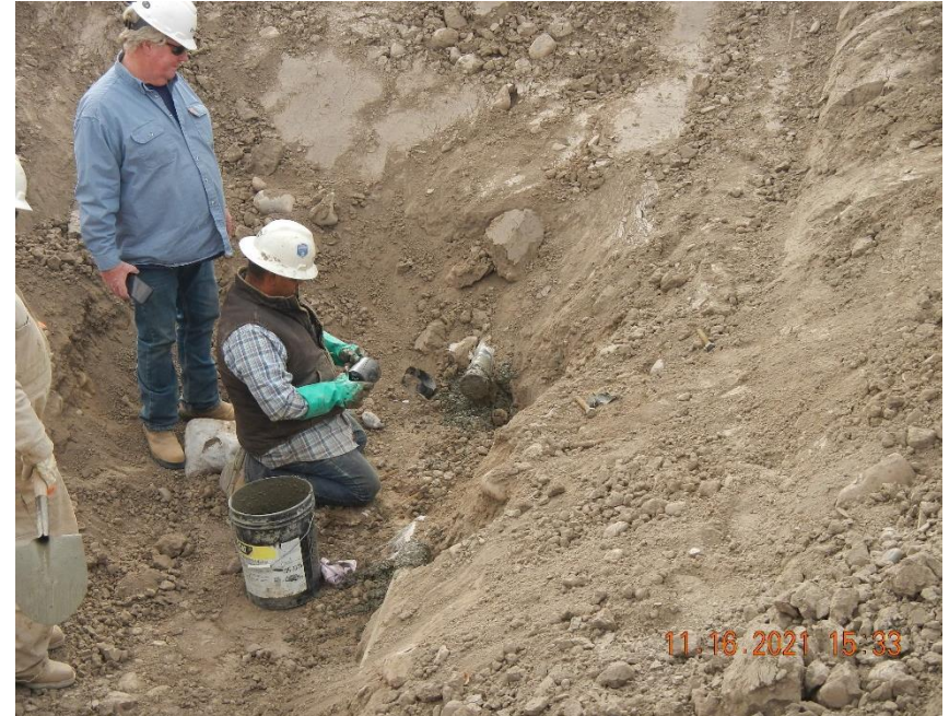
Cementing ends of abandoned flow line.
