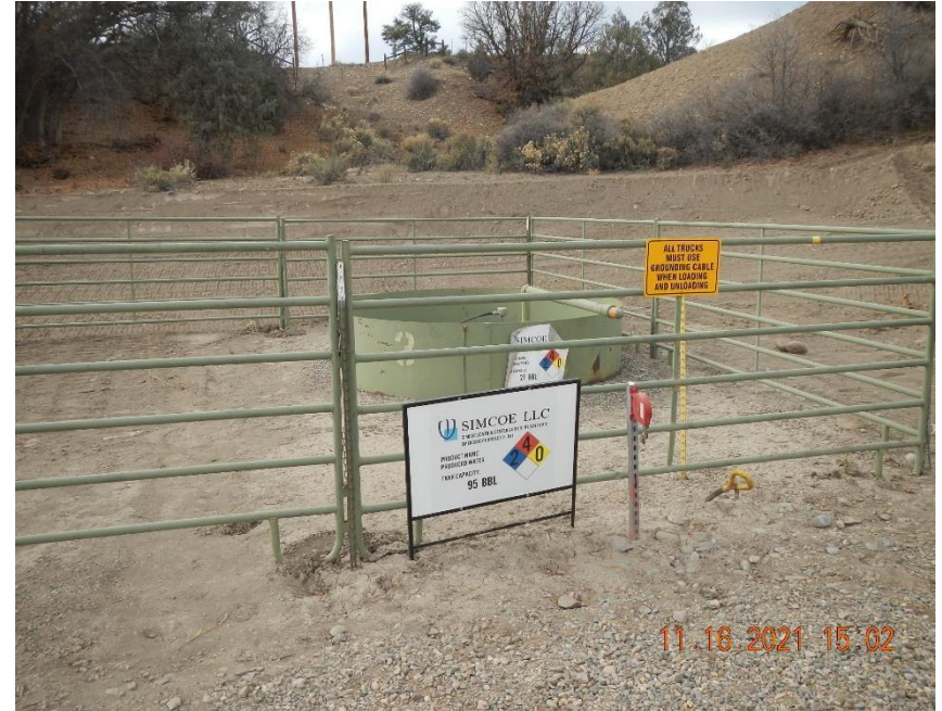
Free standing sign lists capacity as 95 bbl. Sticker lists capacity as 21 bbl.
