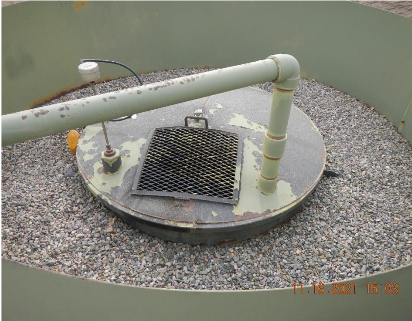
Paint has peeled off of the top of the PBV.
