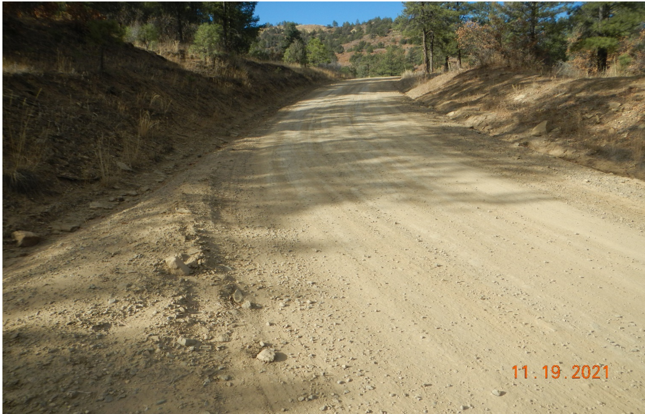
Photo 3. Facing west at the switch back of the road where there was vehicle rutting. The road was graded however, the road was not stabilized and vehicle rutting may occur during wet winter condition.
