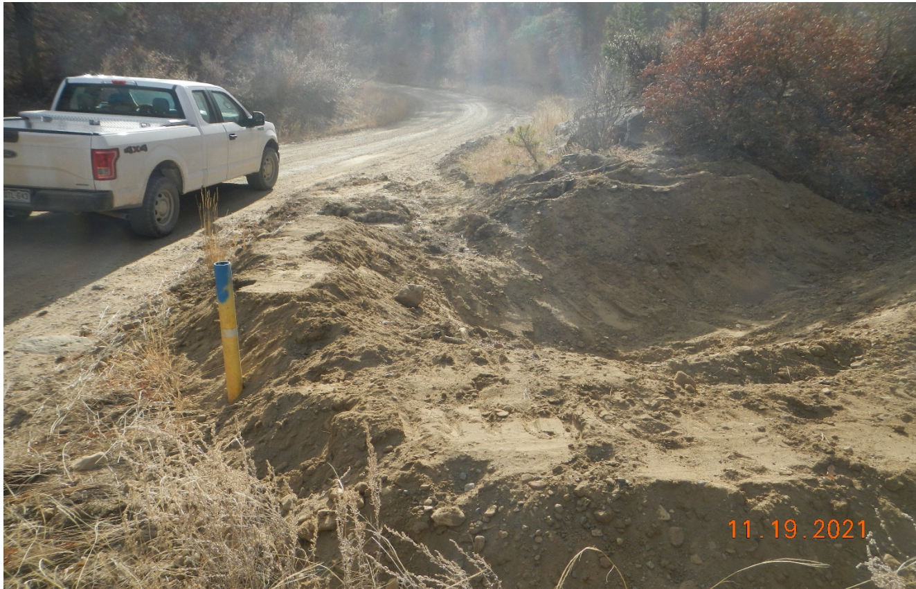
Photo 2. The culvert has been cleaned out. There is sediment piled around the culvert which needs to be reseeded.
