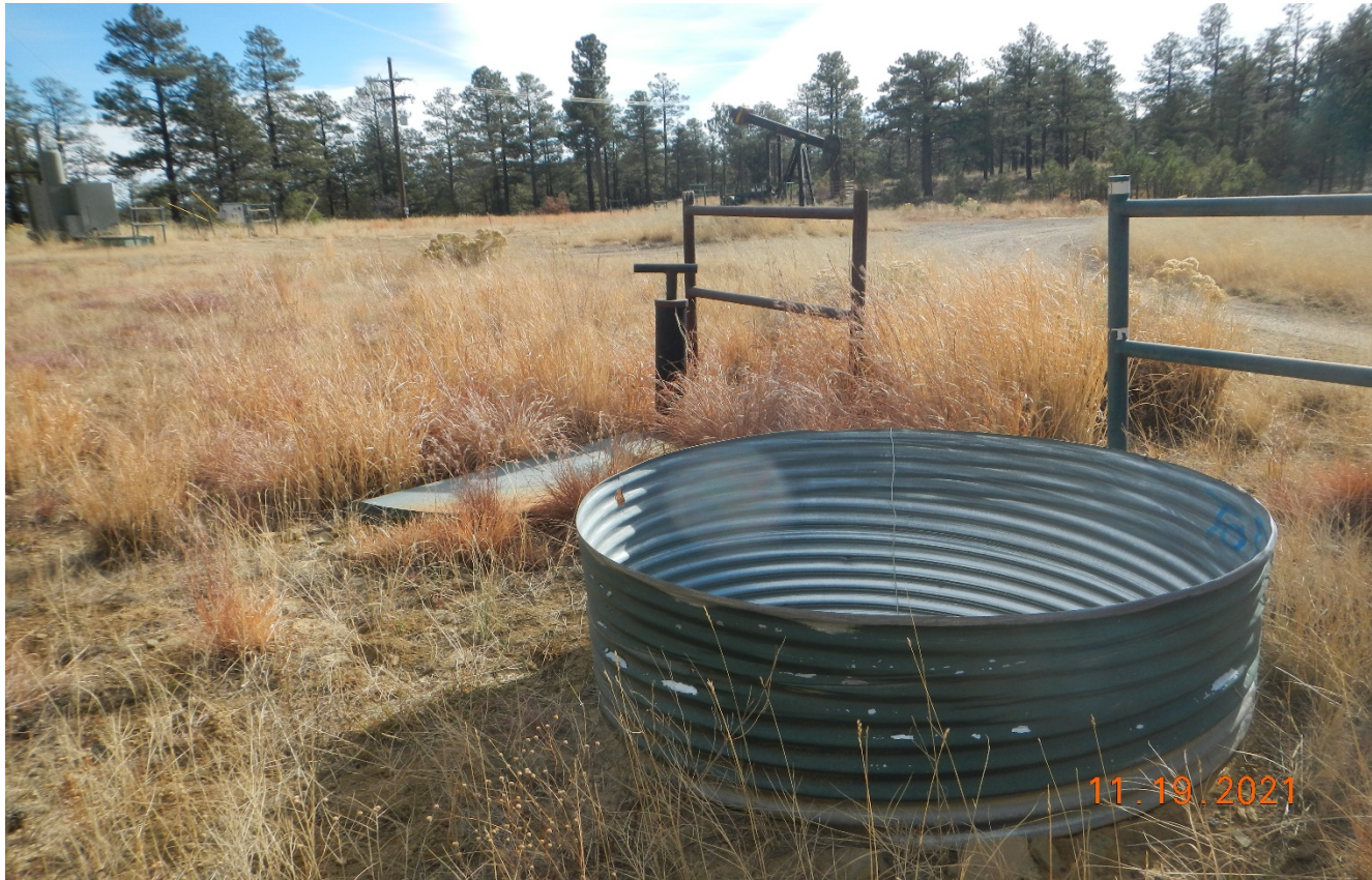
Photo 6. The lid on the culvert needs to be installed to prevent wildlife entry.
