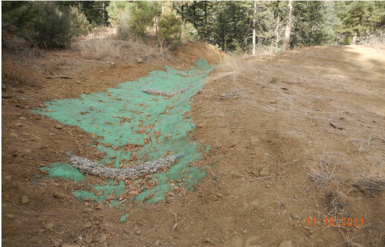
Photo 4. The erosion gully at the second switchback of the road has been reaired and stabilized.
