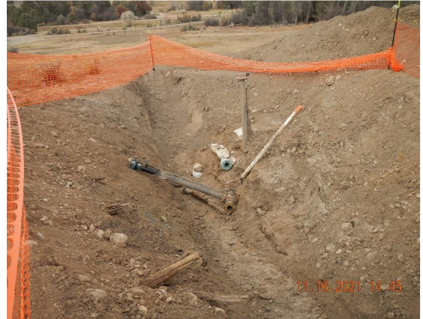
Excavation to expose flow lines being decommissioned as part of REM #20366.
