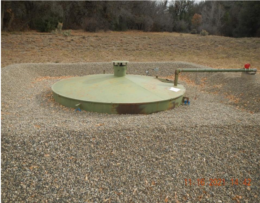
PBV does not have labels as required by Rule 605.h.
