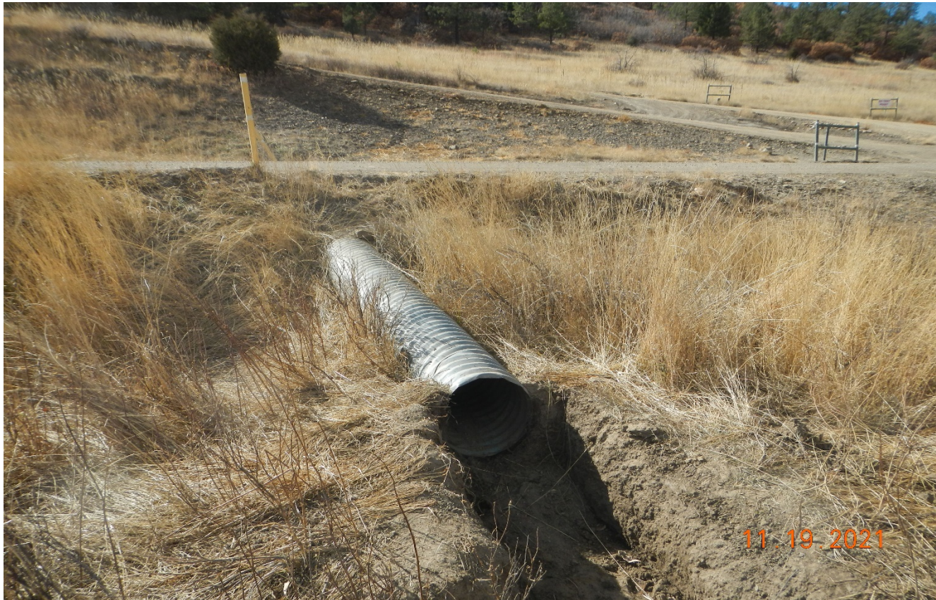
Photo 2. The culvert near the location has been cleaned out and repaired.
