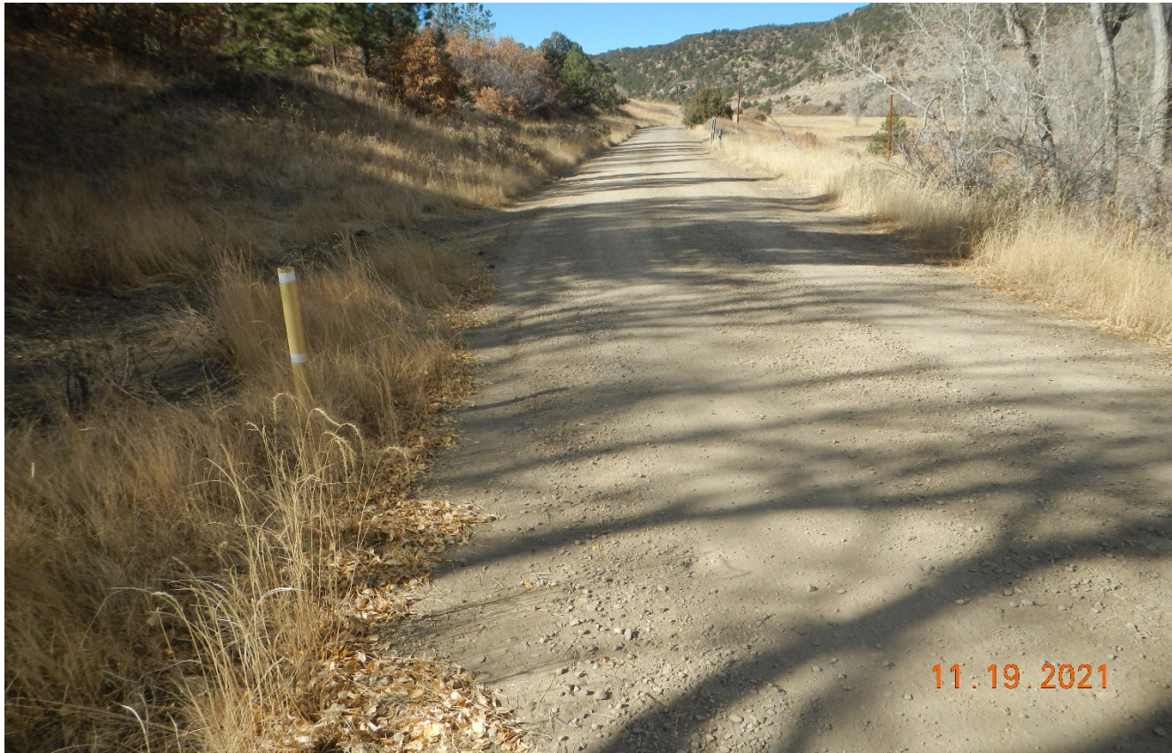
Photo 1. The road was regraded and additional gravel was spread along areas of the road.
