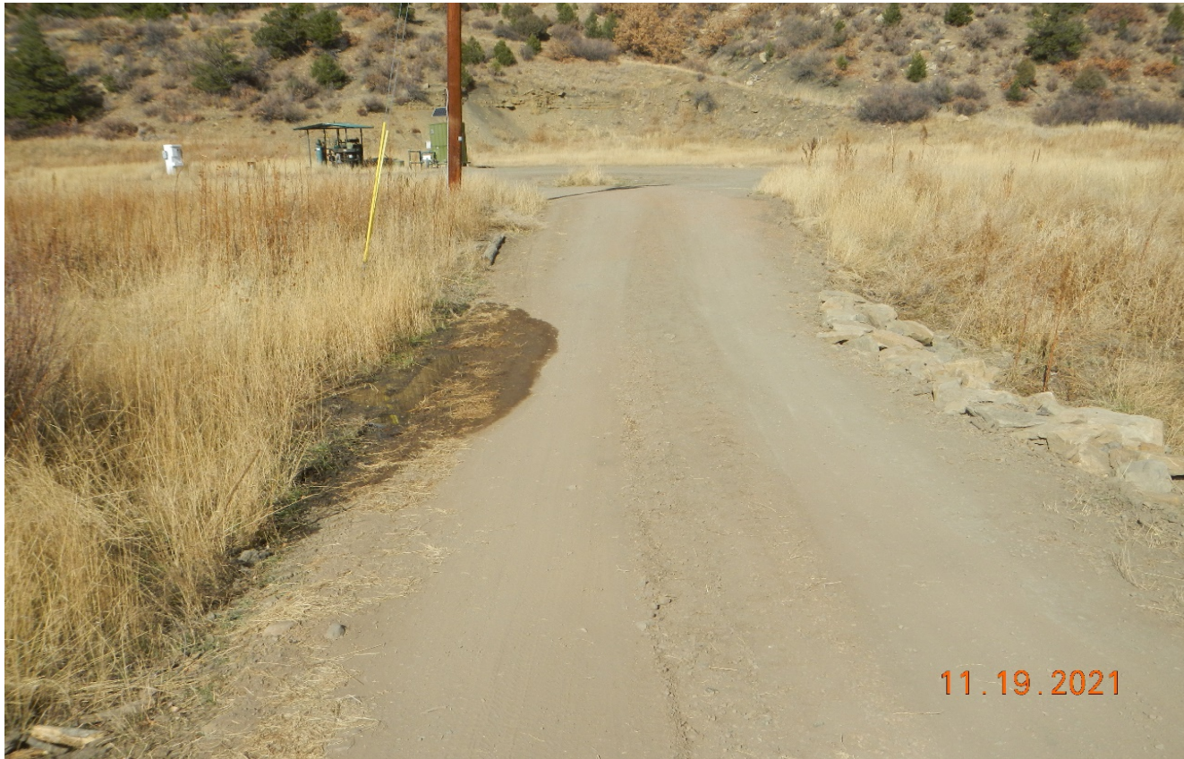
Photo 4. Facing northwest along the access road. This area of the road was repaired. There is water seeping near the road due to a beaver dam upstream. This area may need to be reconstructed to allow water flow during high stream flow periods (e.g. culvert).
