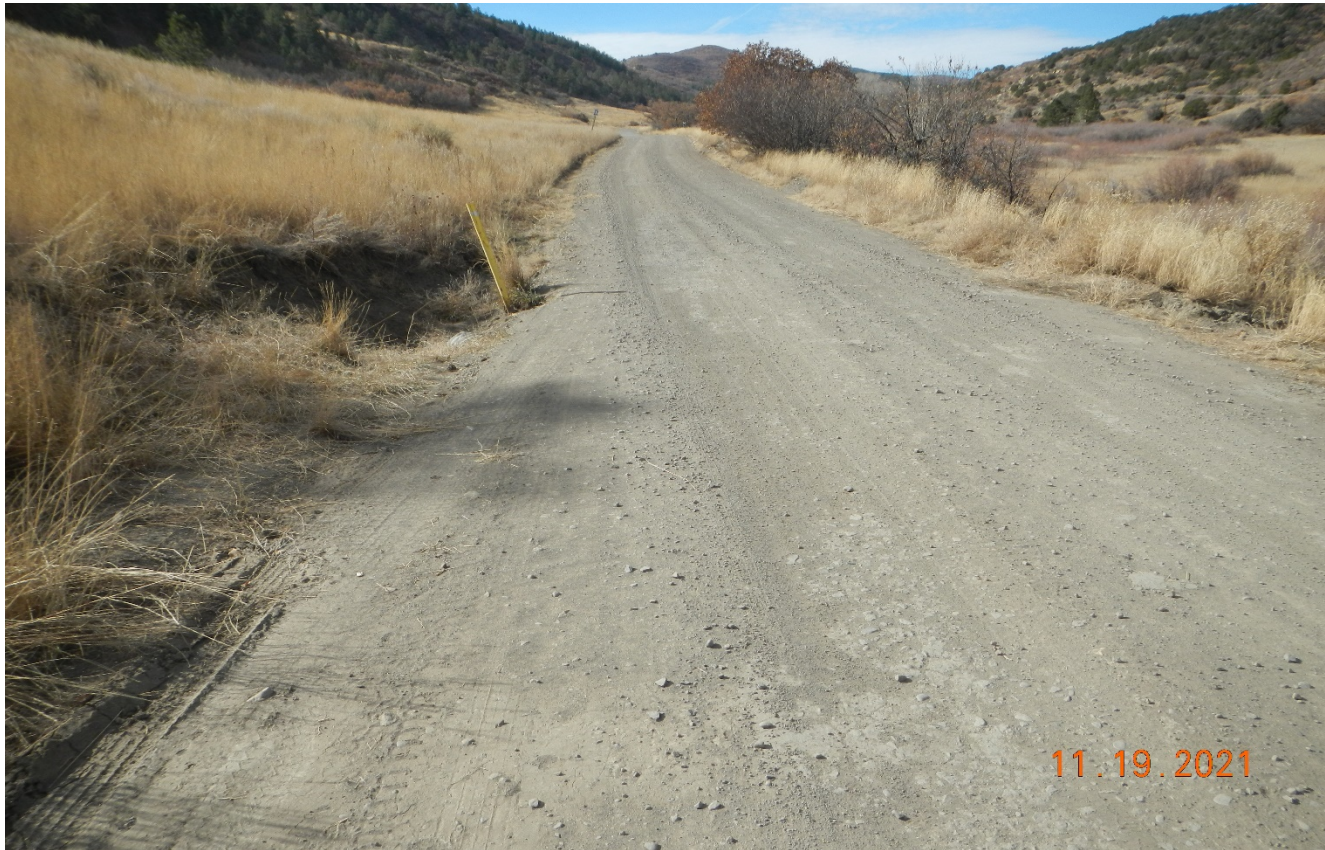
Photo 3. Facing southwest. The road was regraded and additional gravel was spread along areas of the road.
