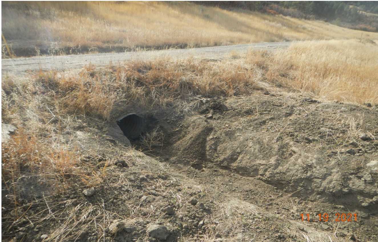
Photo 2. The culverts along the main road have been cleaned out and repaired.
