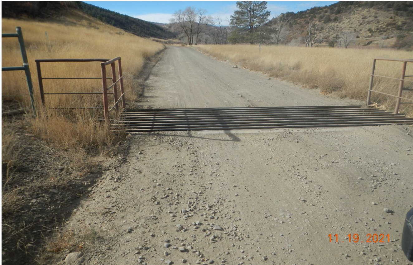
Photo 1. The cattle guard along the main road near the Bingham campground has been repaired.
