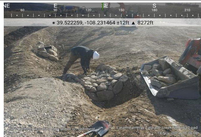
Installing Rock Apron on the Cascade Creek 697-16A2 Pad
