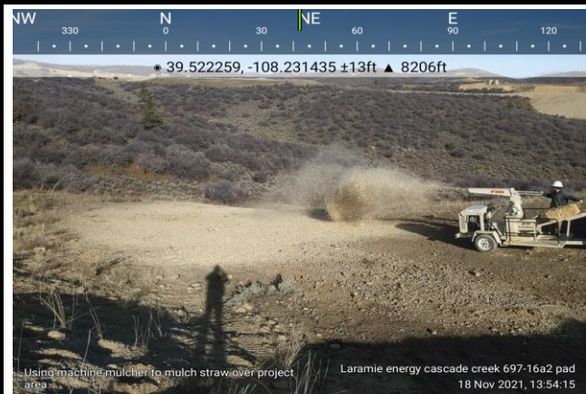
Applying Straw Mulch on Cascade Creek 697-16A2 Pad
