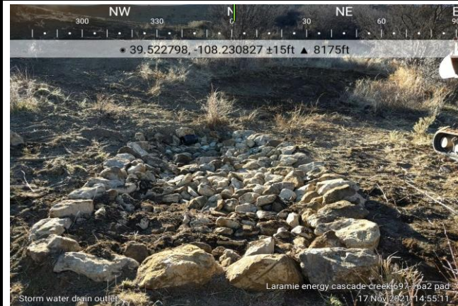
Flex Pipe Outlet and Rock Apron on Cascade Creek 697-16A2 Pad
