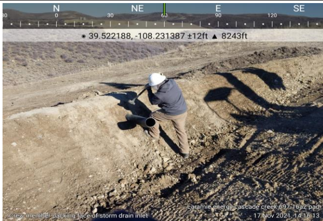
Packing Inlet Flex Hose Face to Create Positive Seal on Cascade Creek 697-16A2 Pad
