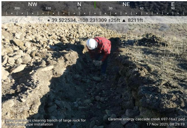
Removing Larger Rock from the Bottom of the Excavation by Hand
