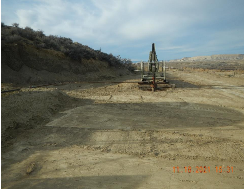
Dead weed debris cleared from location.
