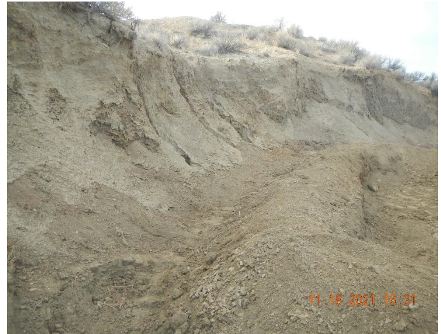
Sediment removed from between cutslope and tank berm.
