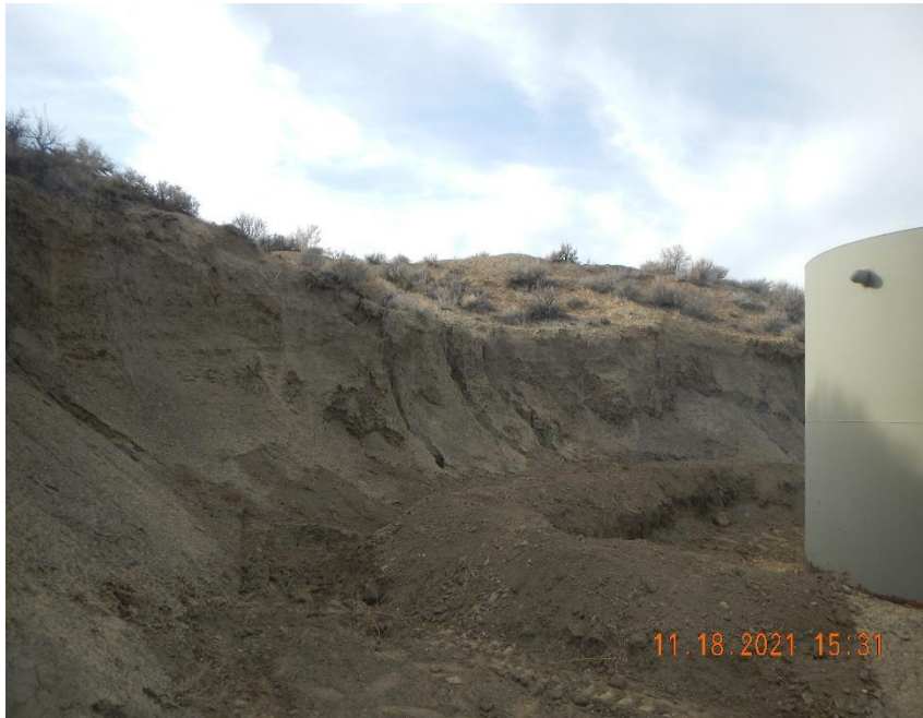
Sediment removed from between cutslope and tank berm.
