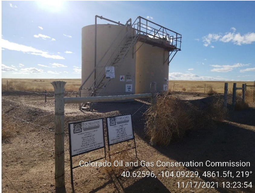
Photo 1 – Tank Battery
