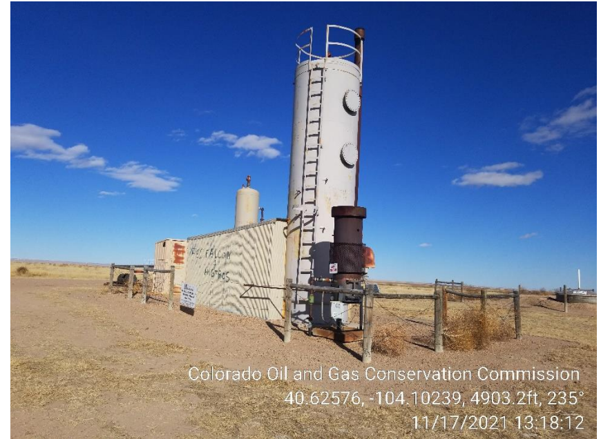
Photo 2 – Heater Treater
