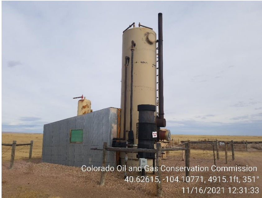
Photo 3 – Heater Treater and ECD
