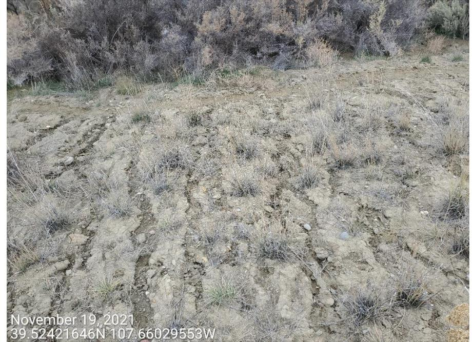
**Photo 3:** Photos taken from the fill slopes along the west end of the Location. Unable to find evidence that work was conducted to address stormwater and erosion degradation issues at the slopes on the west end of the Location. Control measures to manage runoff, and to protect and stabilize slopes of the Location remain missing or insufficient.
