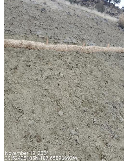
**Photo 2:** Photos taken from the cut slopes along the east end of the Location. Photos provide example showing Operator has placed a single row of straw wattle along portions of the cut slope. Soils along cut slopes remain loose and unstabilized. Control measures to manage runoff, and to protect and stabilize slopes of the Location remain missing or insufficient.
