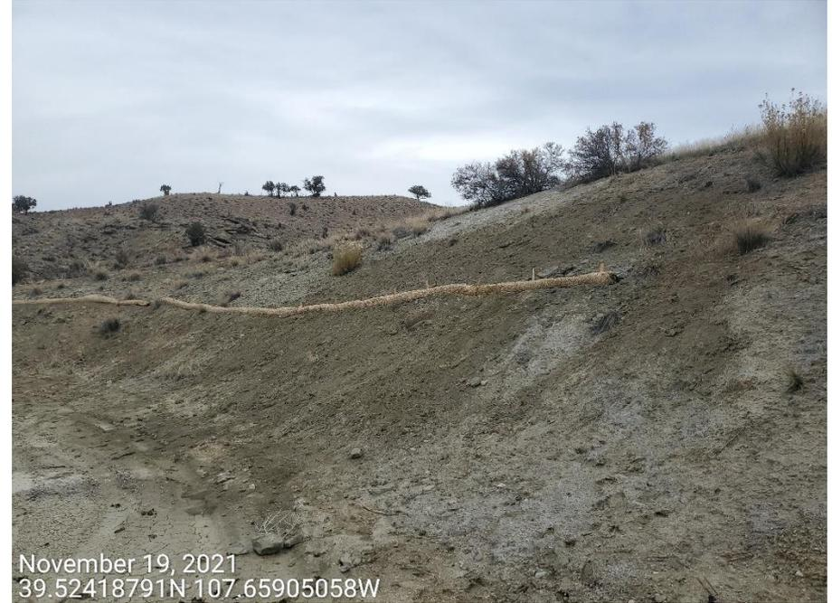
**Photo 1:** Photos taken from the cut slopes along the east end of the Location. Photos provide example showing Operator has placed a single row of straw wattle along portions of the cut slope. Soils along cut slopes remain loose and unstabilized. Control measures to manage runoff, and to protect and stabilize slopes of the Location remain missing or insufficient.
