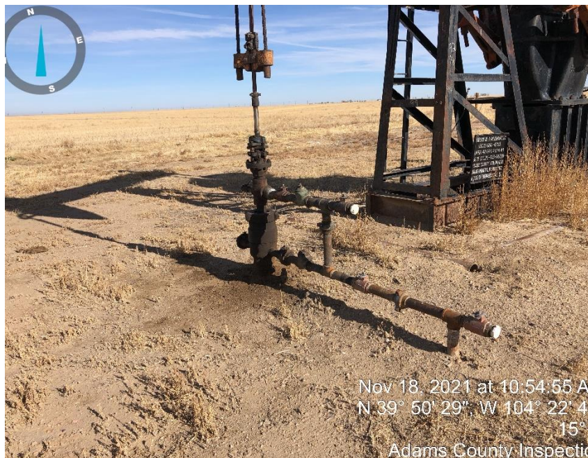
Photo #4 stained soil around well head.
