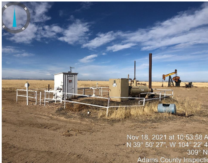
Photo #2 separator and meter.
