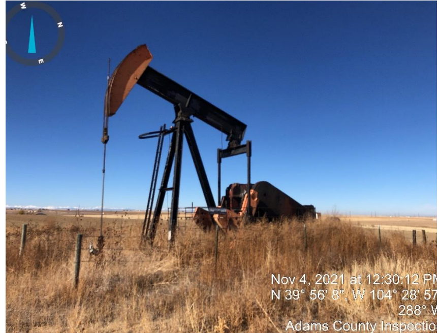
Photo #4 Pump Jack.
