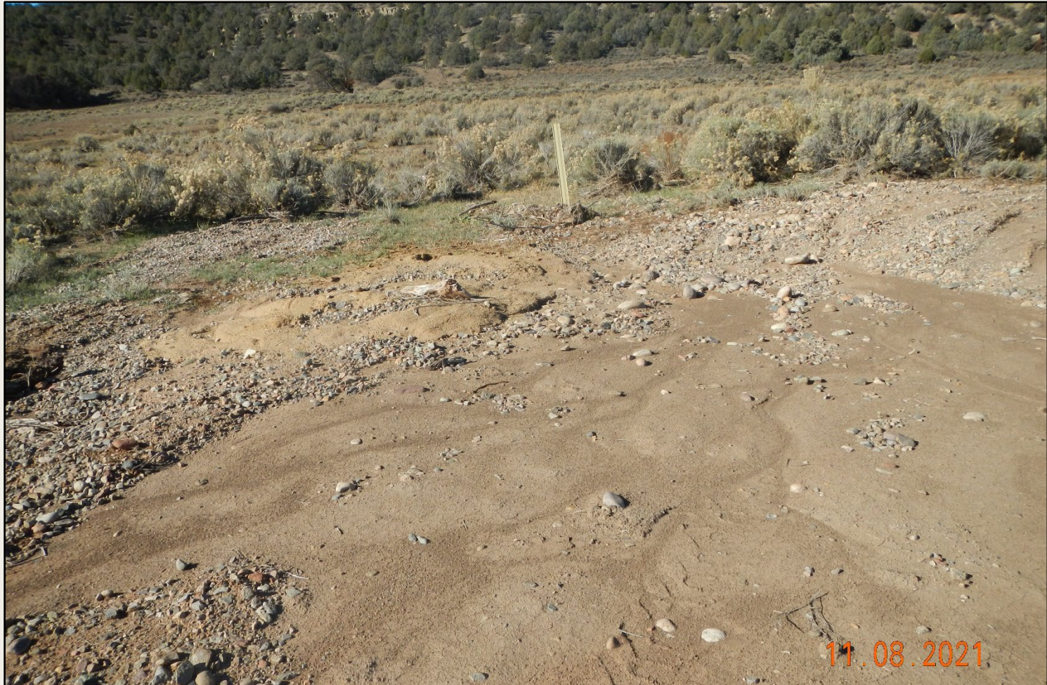
Photo 5. View of the southern project area, where gravel is washed down-slope and off of the well pad. Bare soils are scoured.
