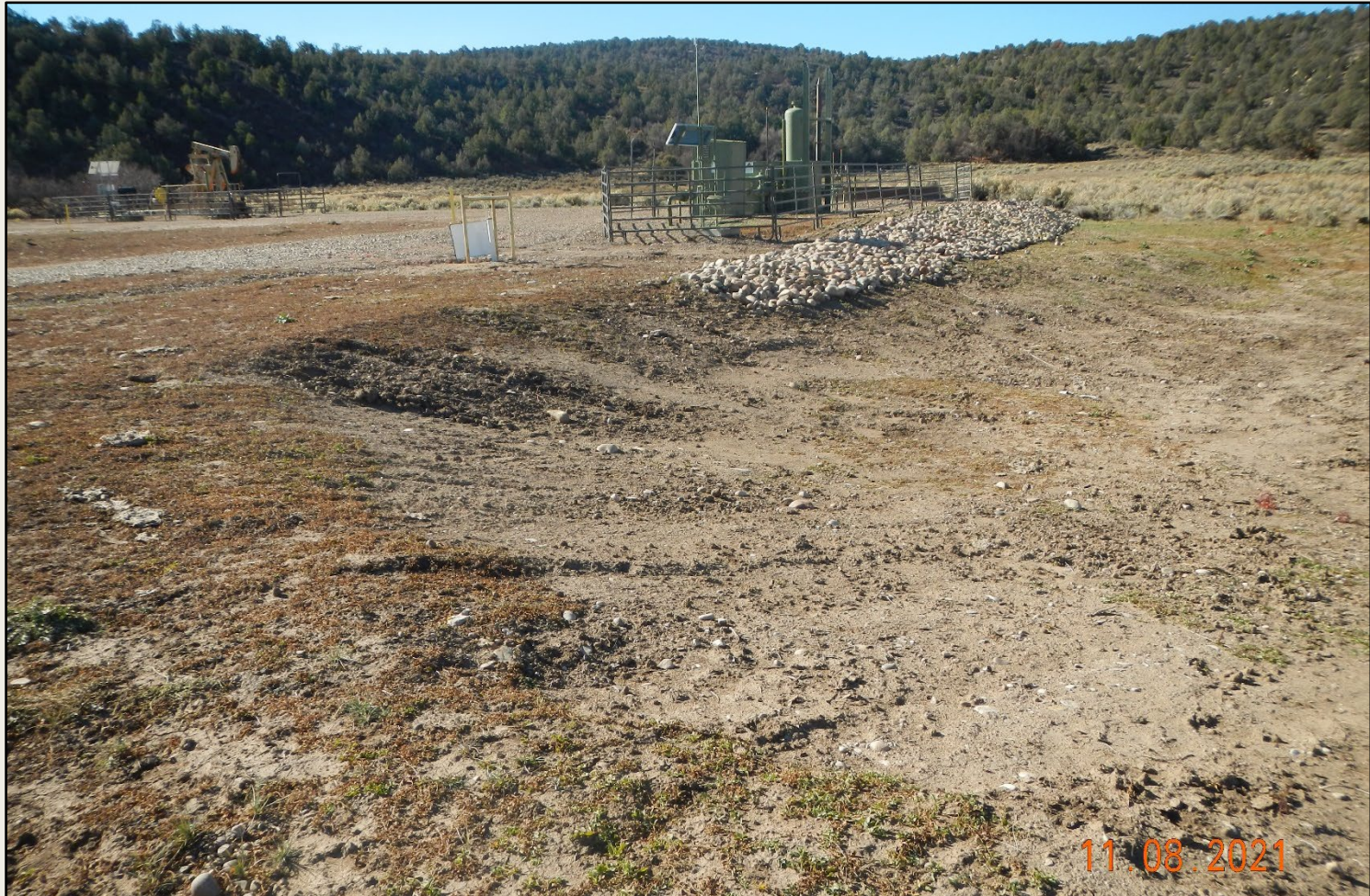
Photo 4. View of the western project area. Eroded areas are recontoured and cobbles placed on western (downstream) edge of facilities area. Cobbles are approximately 4-6 inches in diameter are not adequately sized to prevent erosion.
