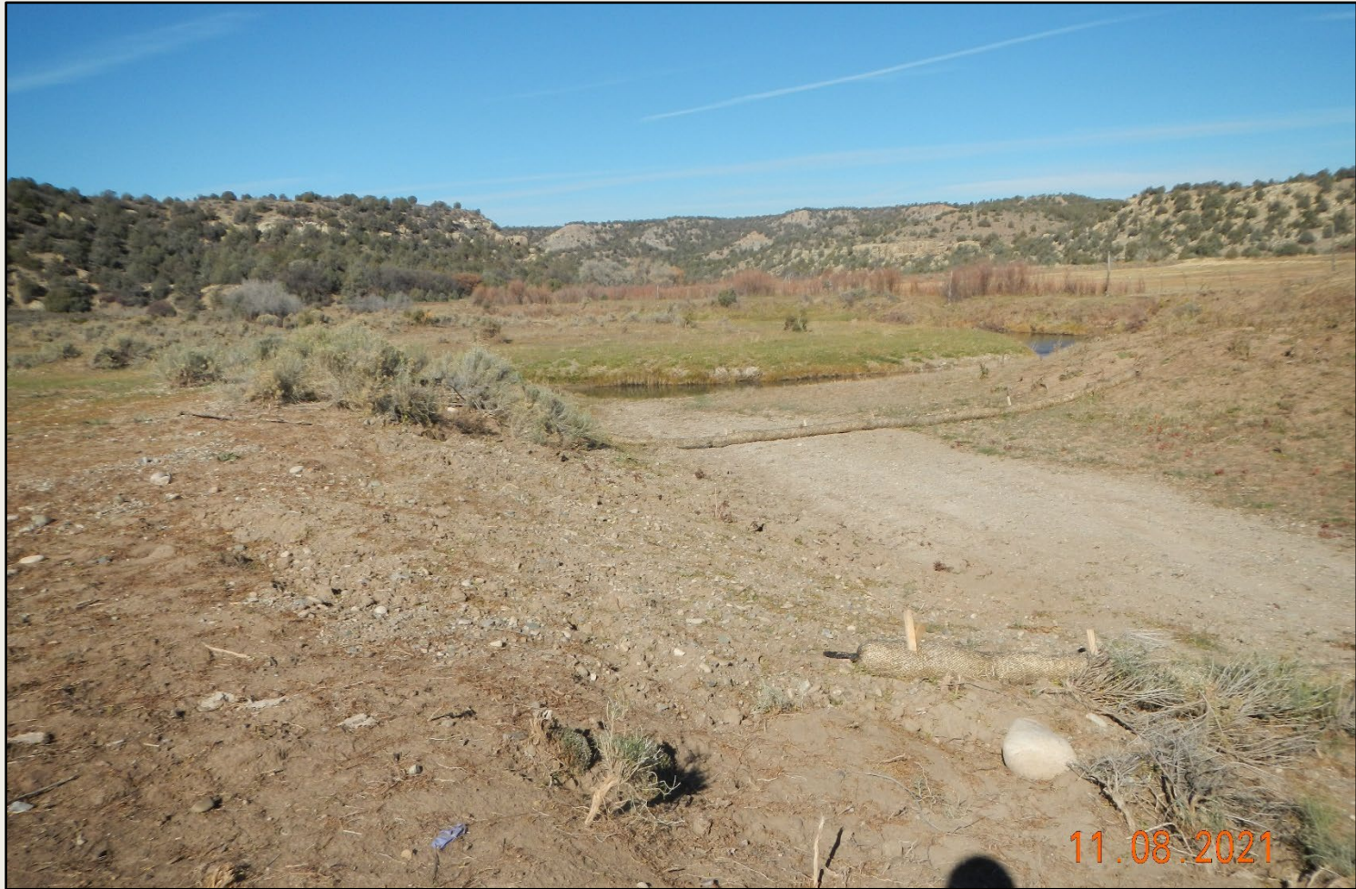
Photo 3. View of swale north of the well pad; gravel removed and wattles installed. Reseeding and stabilization not conducted on scoured soils. Wattle is not a appropriate stormwater control for this area.
