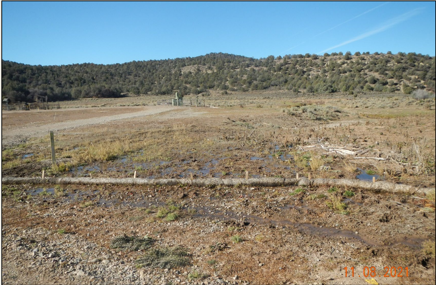
Photo 2. View of straw wattle in the northern project area. This is not an appropriate stormwater control for this area. Wattles are not properly installed.
