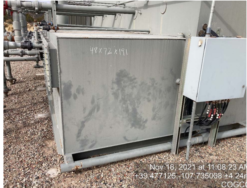
Glycol vessel lacking labeling/dimensions
