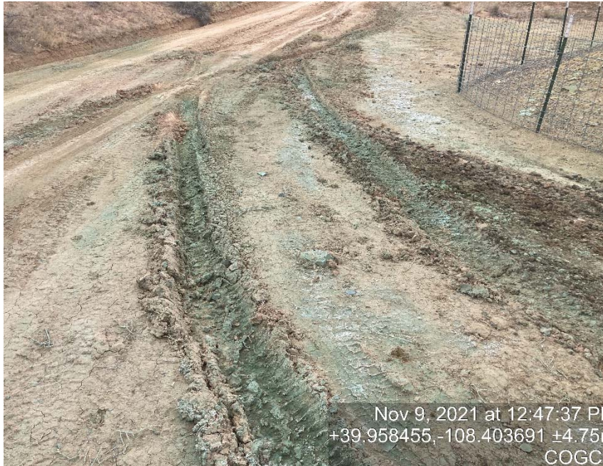
Lack of stabilization/compaction
