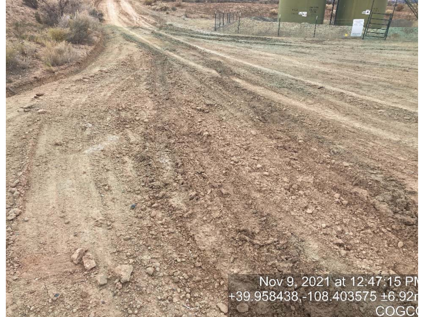
Lack of stabilization/compaction
