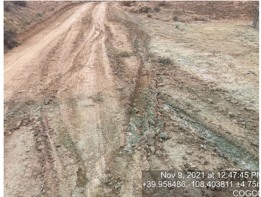
Lack of stabilization/compaction
