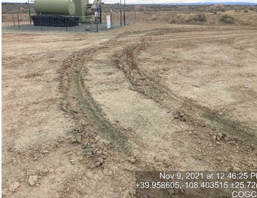
Lack of stabilization/compaction
