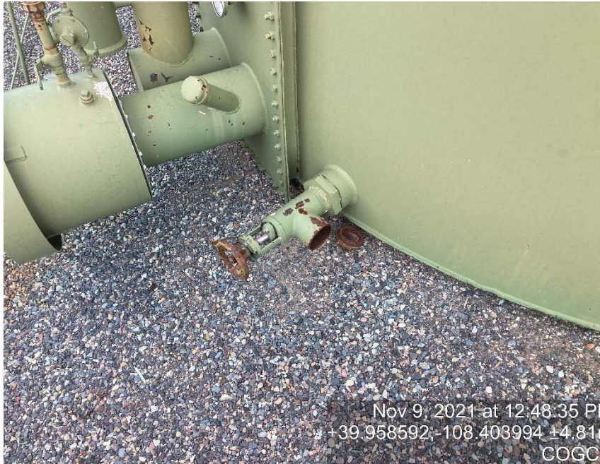
Load out line missing bull plugs/caps
