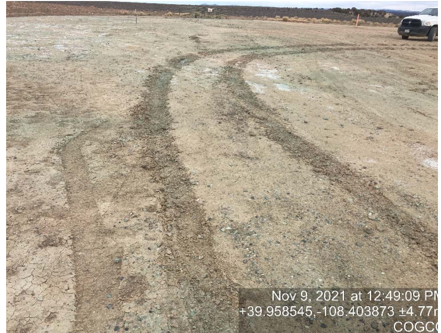
Lack of stabilization/compaction
