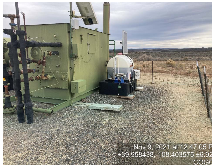
Glycol vessel lacking labeling
