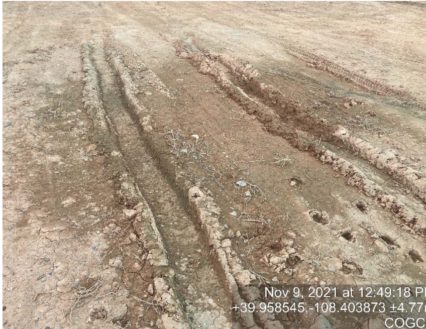
Lack of stabilization/compaction
