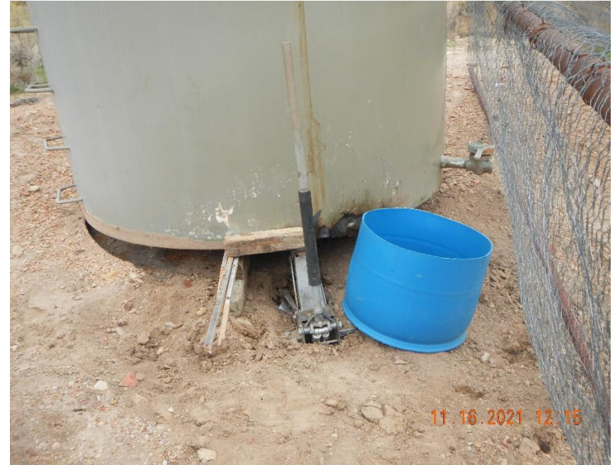
Tank has been lifted for repair and inspection.
