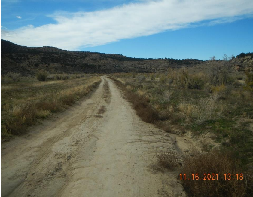
Erosion and rutting on road.
