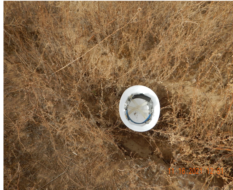
Photo 8. Photo taken along what is believed to be a flowline, illustrating subsidence. Subsidence was observed throughout the majority of the flowline.
