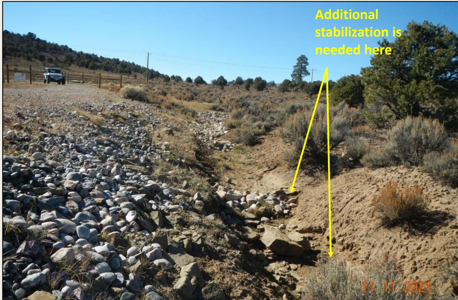
Photo 3. View of stormwater controls installed within the western project area. Additional stabilization is needed in the northwestern portion of the project area where erosion continues around rock check.
