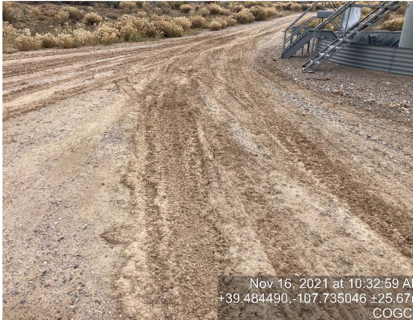
Lack of stabilization/compaction
