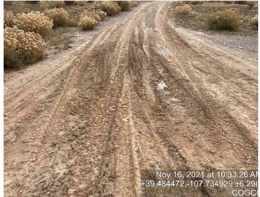
Lack of stabilization/compaction
