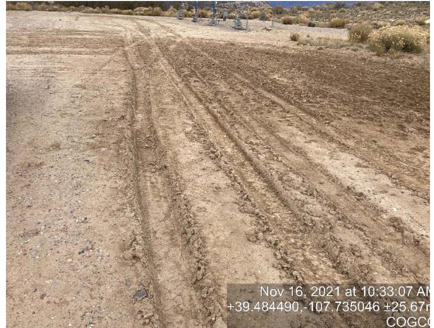
Lack of stabilization/compaction
