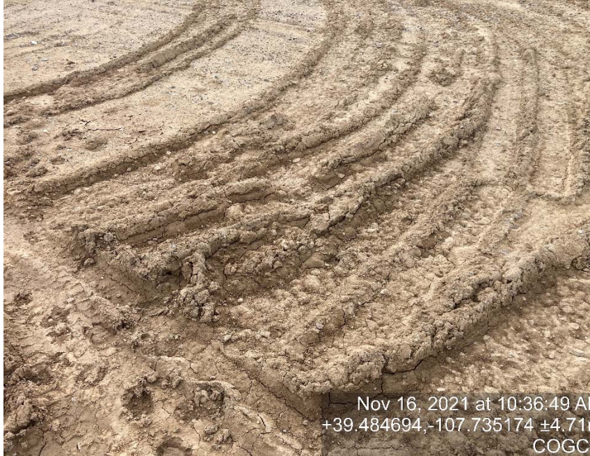
Lack of stabilization/compaction
