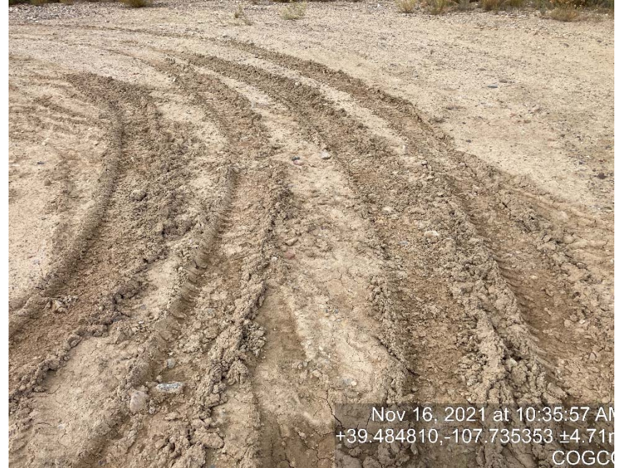
Lack of stabilization/compaction
