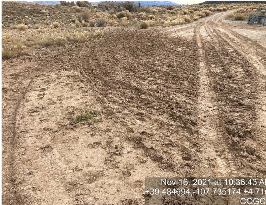
Lack of stabilization/compaction
