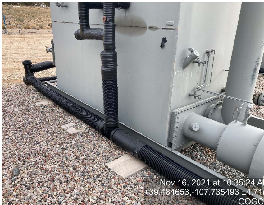
Glycol vessel lacking labeling
