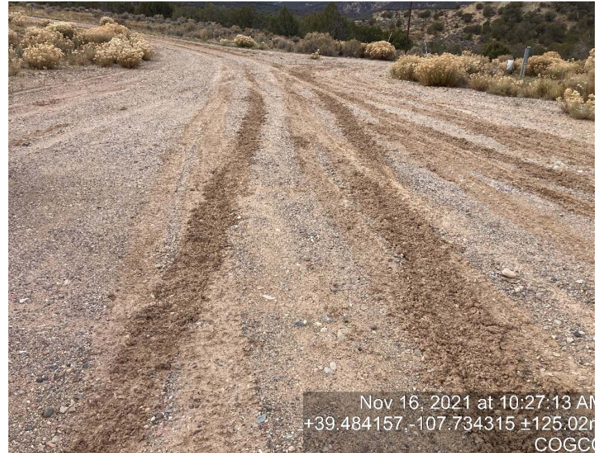
Lack of stabilization/compaction
