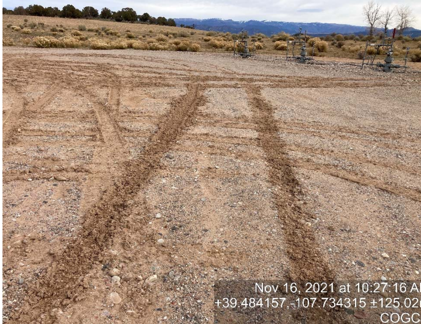
Lack of stabilization/compaction
