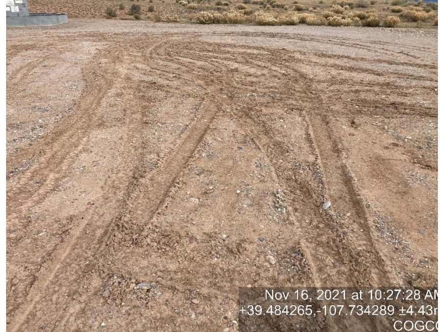
Lack of stabilization/compaction
