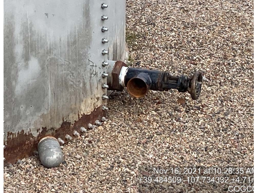
Load out line missing bull plug
