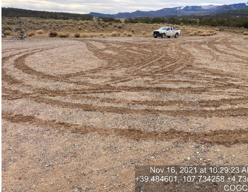
Lack of stabilization/compaction
