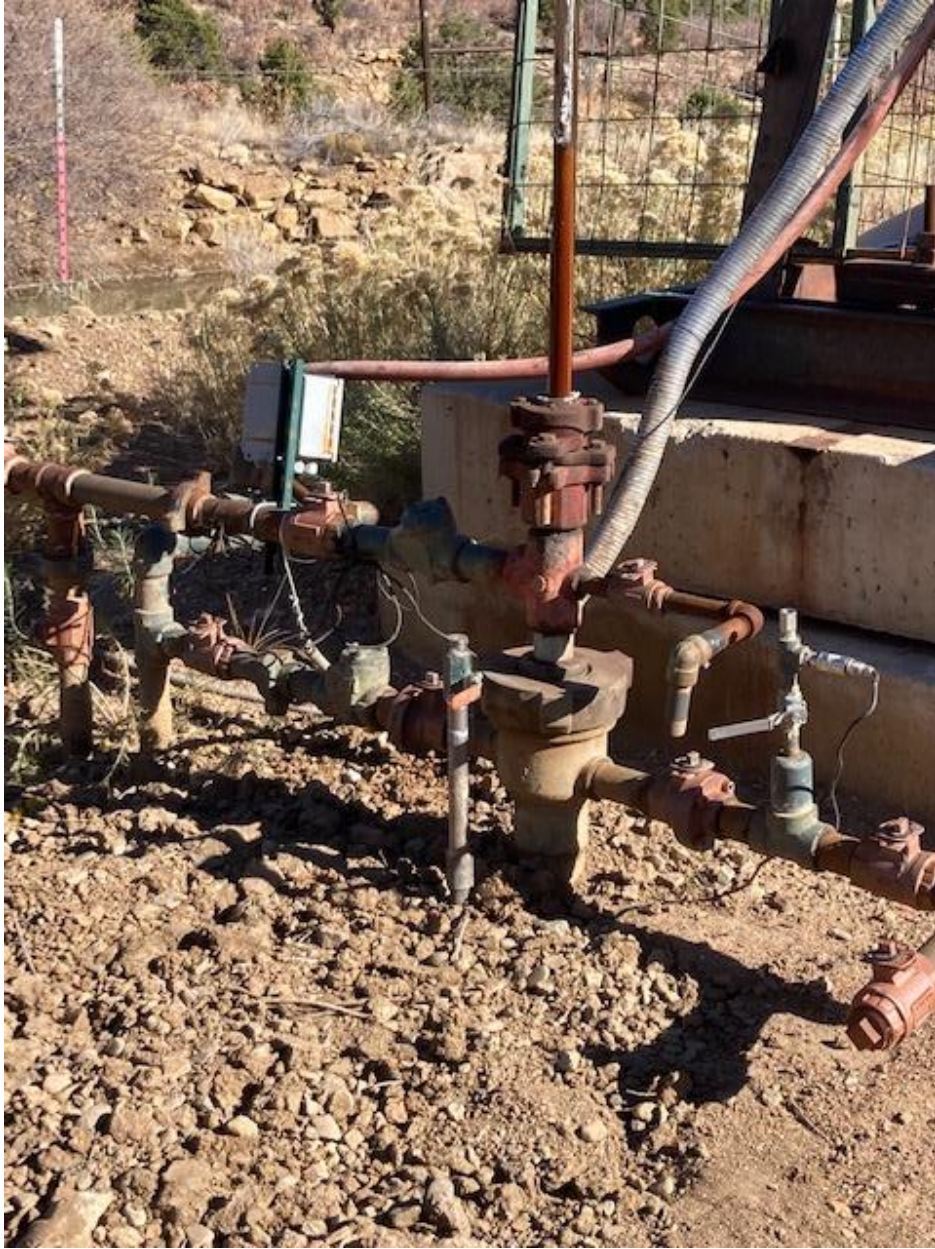
Installed appropriate fittings to allow bradenhead visual inspection as per Rule 419.a
