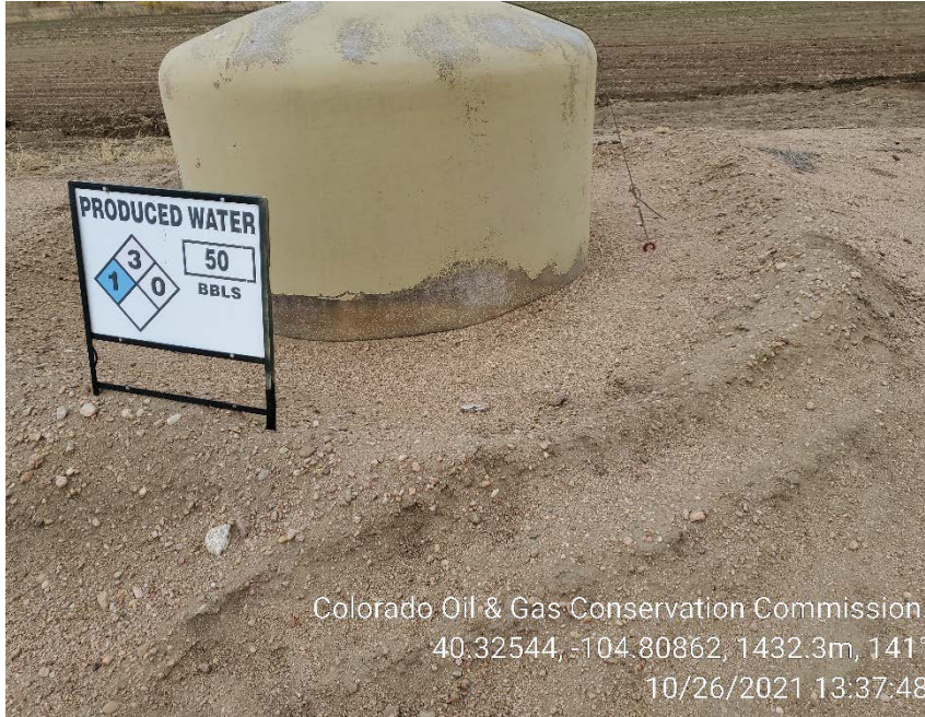
Produced water tank berm on 10/26/2021
