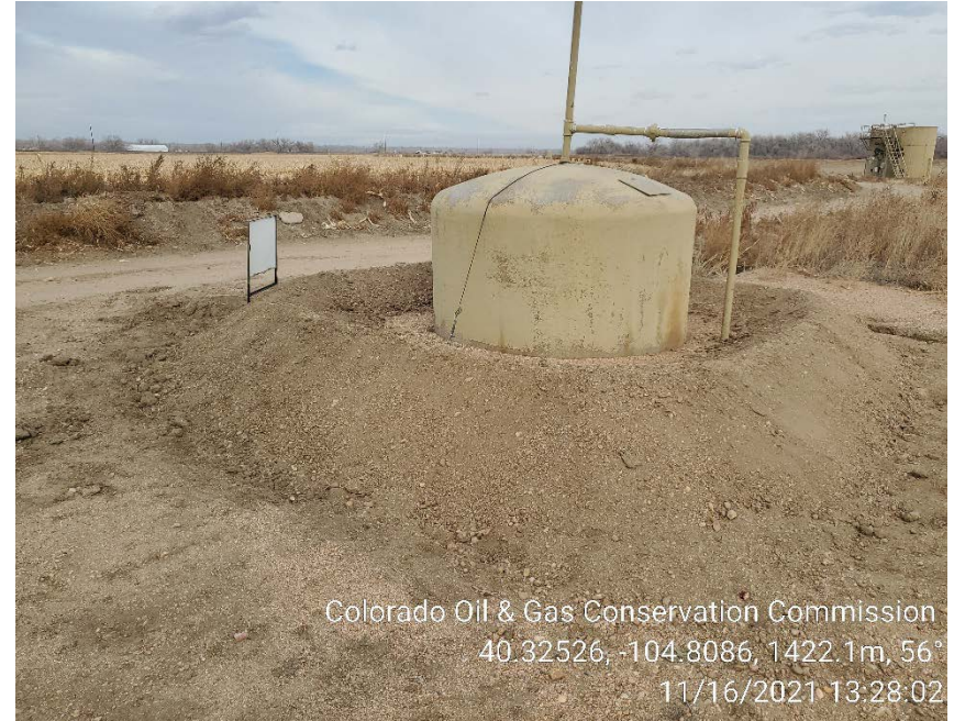
Produced water tank berm on 11/16/2021
