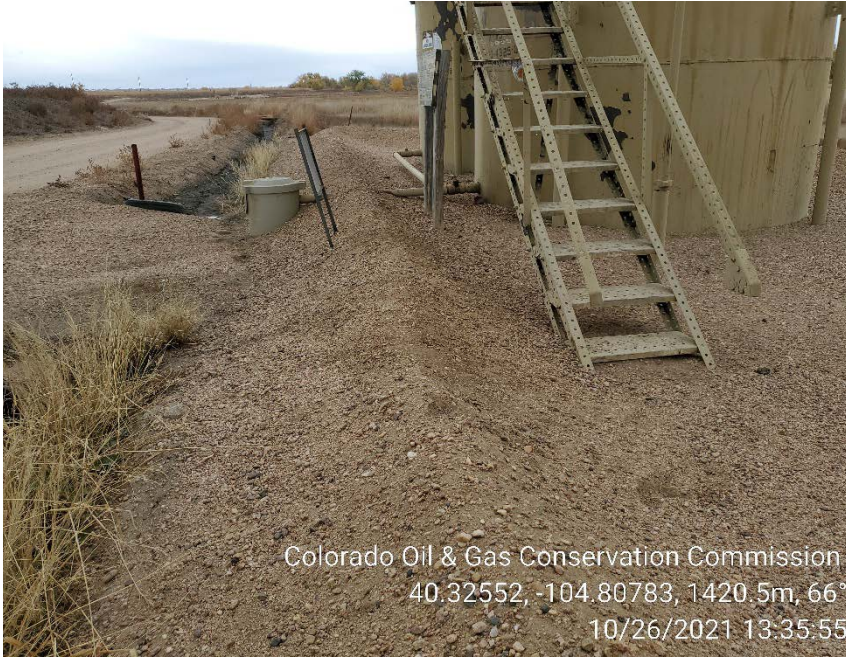
Crude oil tank berm on 10/26/2021
