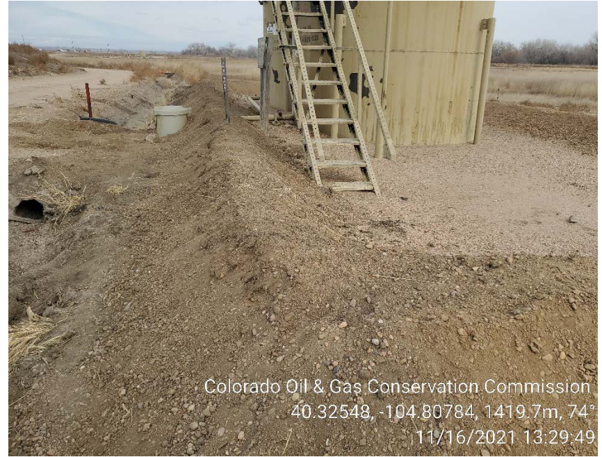
Crude oil tank berm on 11/16/2021
