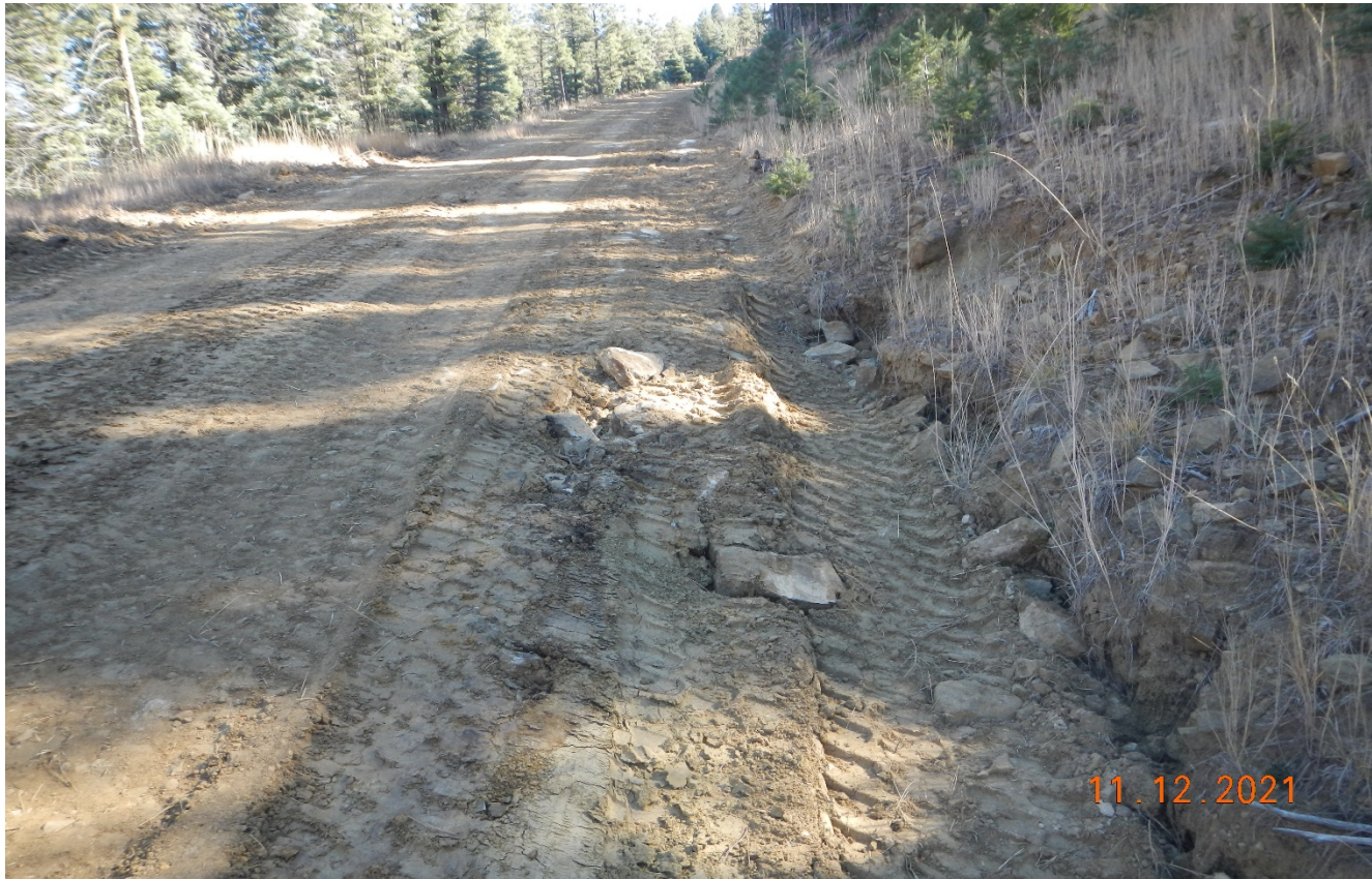
Photo 7. The erosion along the road side was filled but is not stabilized.
