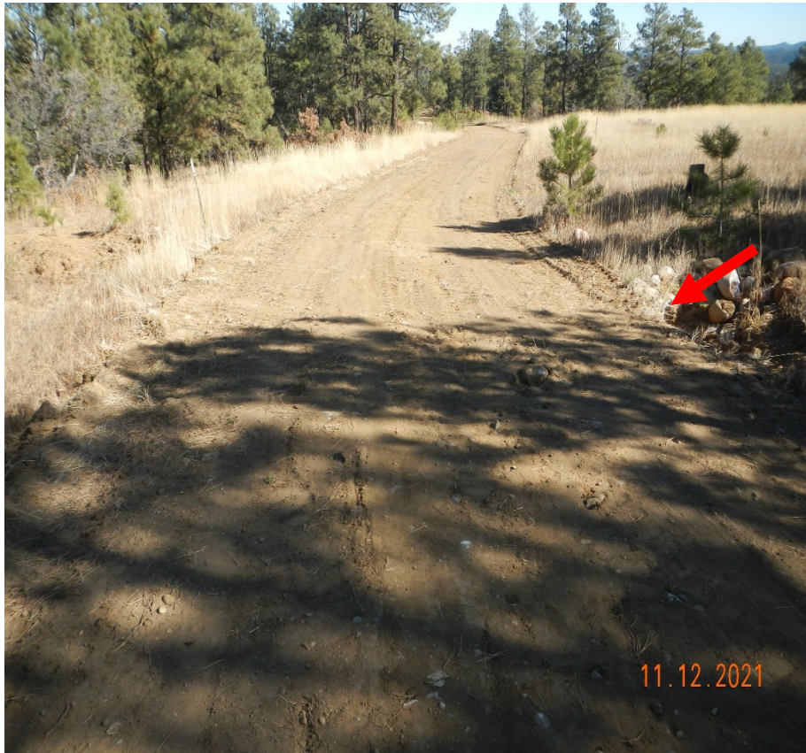
Photo 3. There is a culvert shown at the red arrow which is filled in with sediment.
