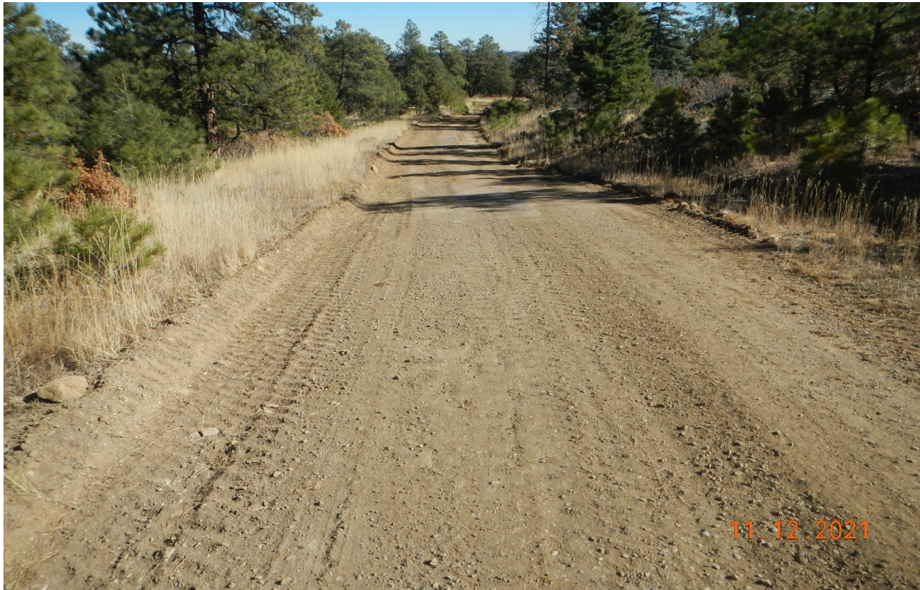
Photo 1. Facing northeast along the access road. The erosion along the road has been graded and repaired..
