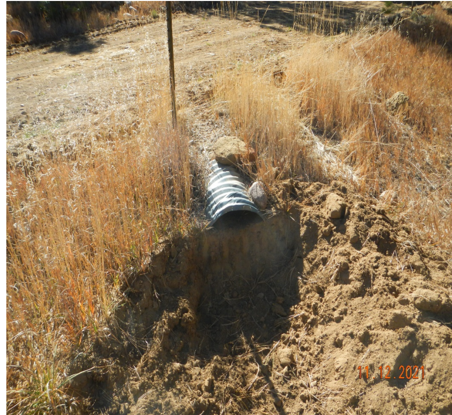
Photo 4. The culvert outlet needs to be cleaned out.
