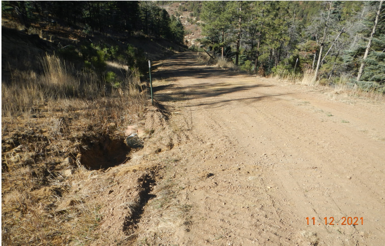
Photo 5. Facing northwest toward road turns down the hill side into the canyon. The culverts have been cleaned out. There is gravel along this portion of the road but further down the road gravel was not observed.
