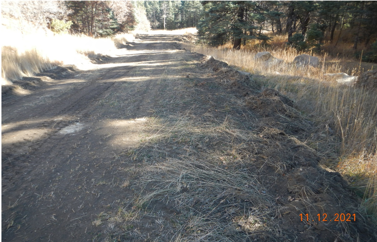
Photo 11. Facing east along the access road. Grading of the road has pushed soil into a row which needs to be raked/leveled out.
