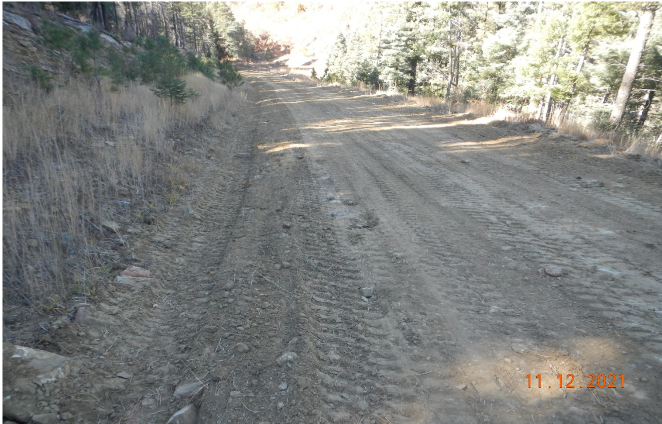
Photo 6. The road was graded down to the canyon bottom and erosion was repaired however there is no insufficient stabilization of the road and road side. There is no gravel along this steep portion of the road.
