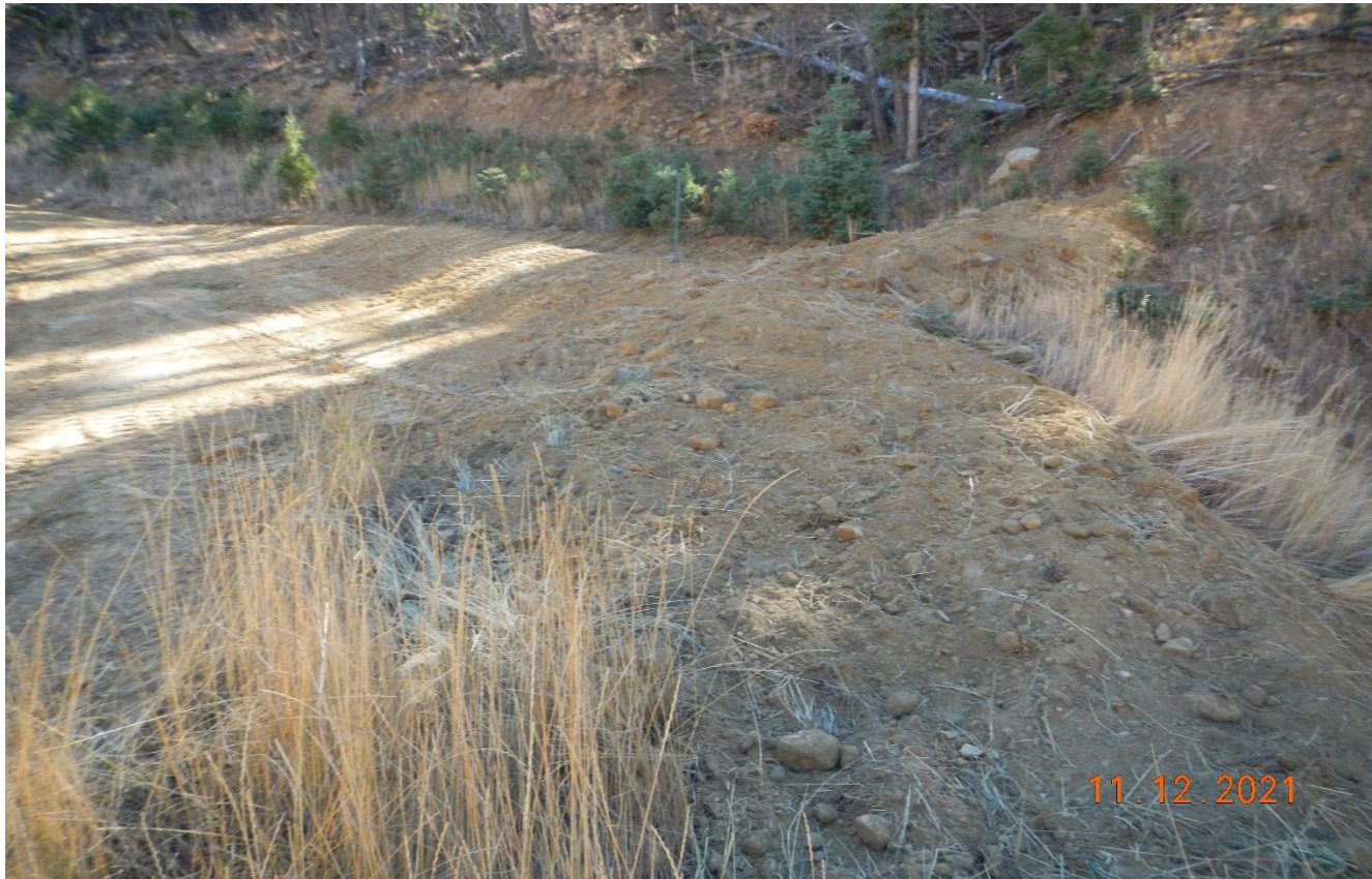
Photo 8. Standing at where road turns at the bottom of the canyon. Disturbed soils have not been seeded and stabilized.
