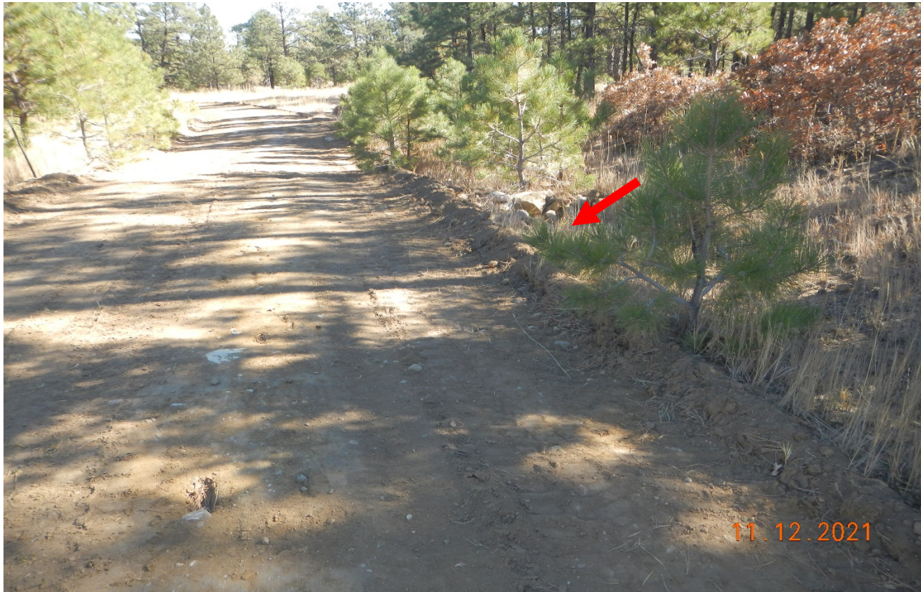
Photo 2. The grading created has pushed dirt into a row which blocks stormwater from flowing toward the culvert shown at red arrow.
