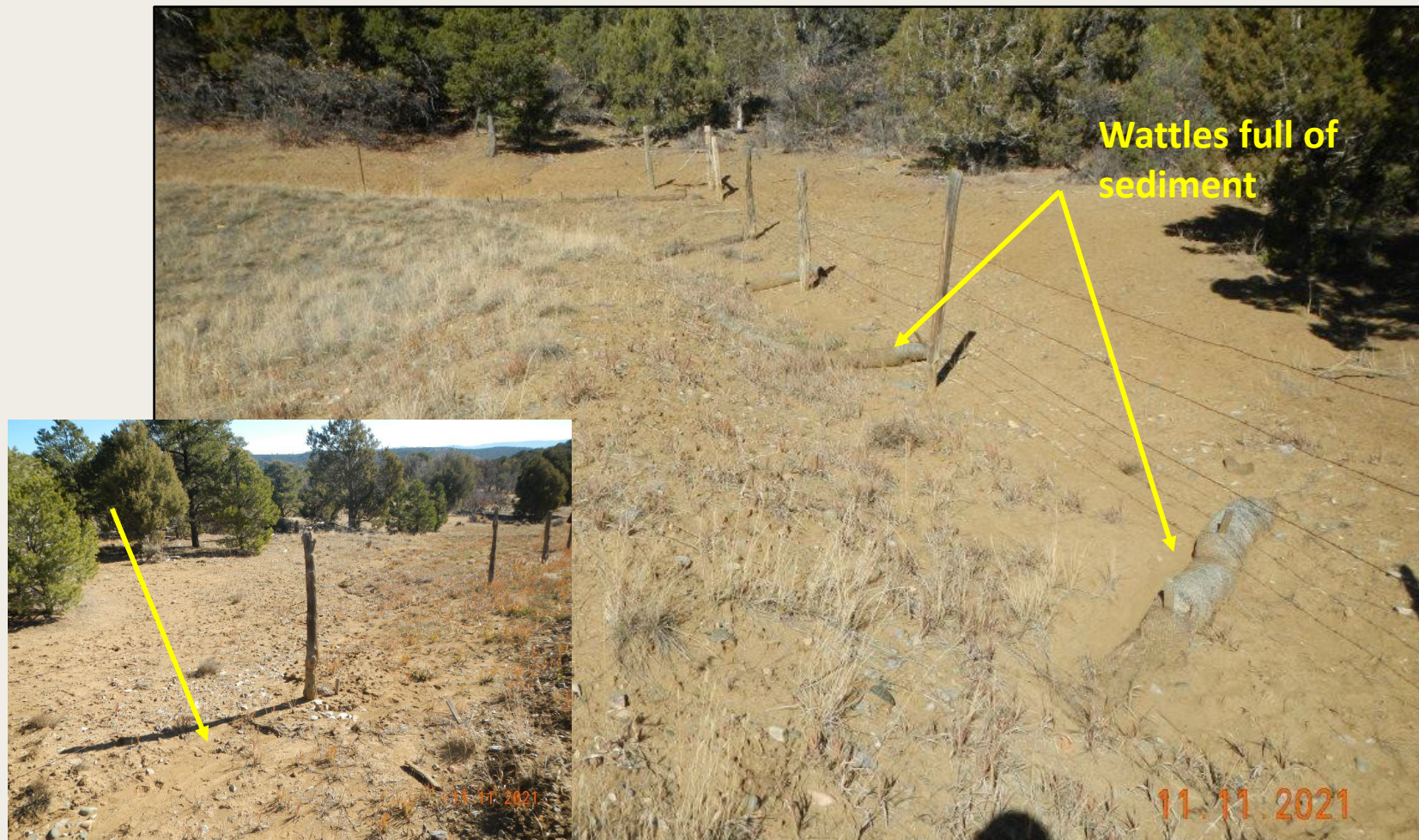
Photo 4. View of straw wattles full of sediment in the northwestern project area. Inset shows erosion downstream from wattles where additional stabilization is needed.
