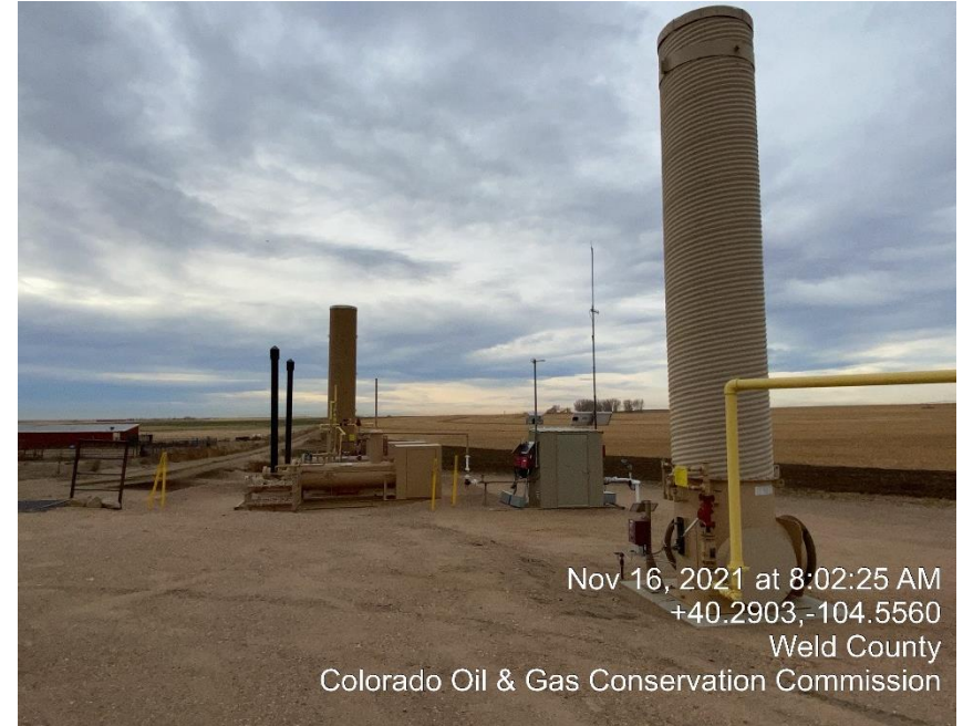
Photo #2 Production Equipment
