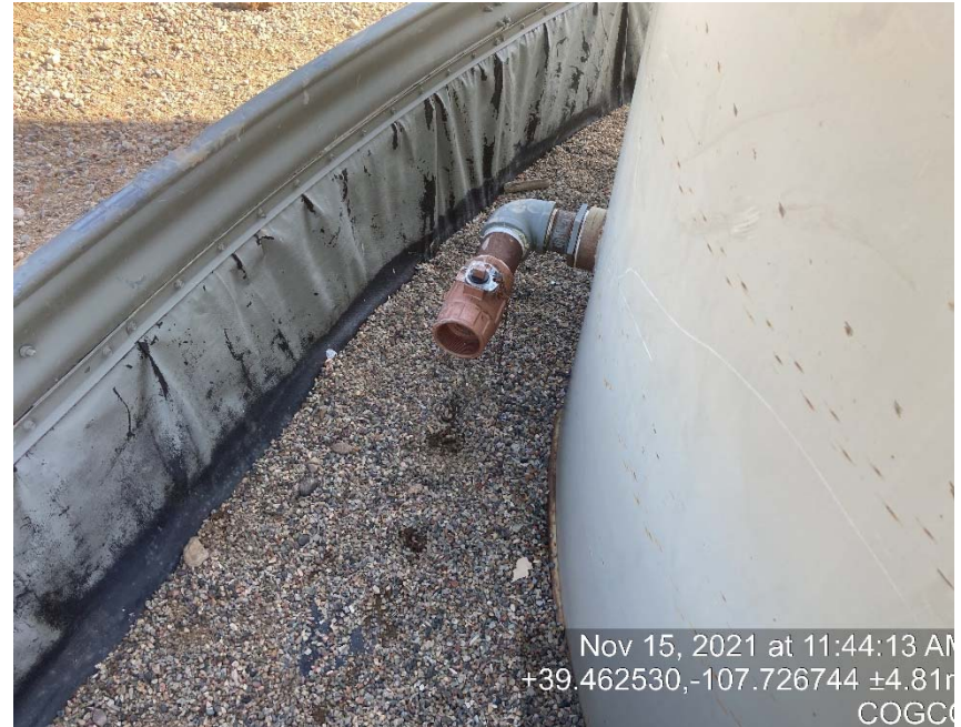
Load out lines lacking bull plugs/caps
