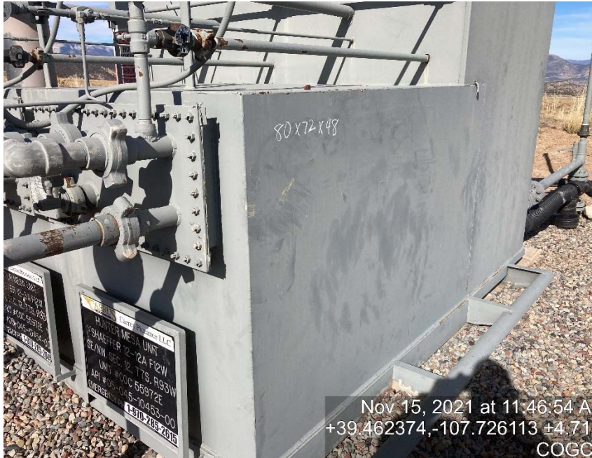
Glycol vessel lacking labeling
