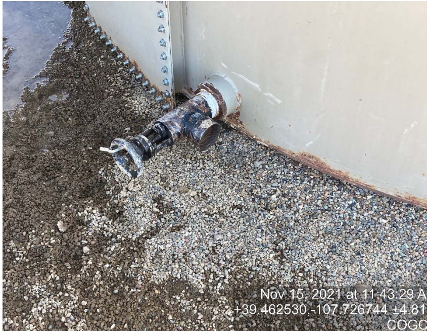
Load out lines lacking bull plugs/caps
